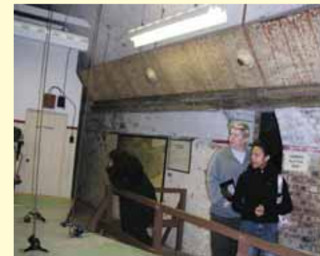
Fig 12 (above) Original ventilation ductwork in tunnel casemate.
