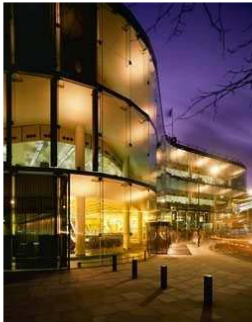
Willis Faber Building Ipswich
