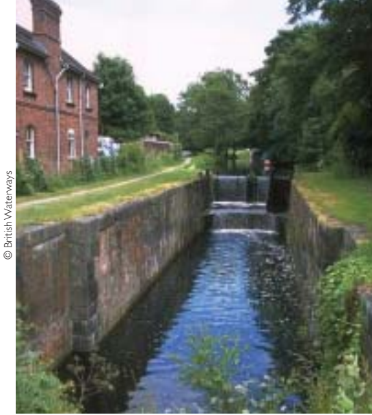
Pike Lock, Stonehouse. Built c. 1777, Pike Lock forms part of the Eastington flight on the Stroudwater Navigation. The chamber is lined in brick, with stone capping and stone quoins to the ends and the gate recesses. It has been restored, but is not working and water is held back by a dam at the top end of the lock
