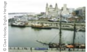
The Liverpool waterfront, looking north west from the Albert Dock
