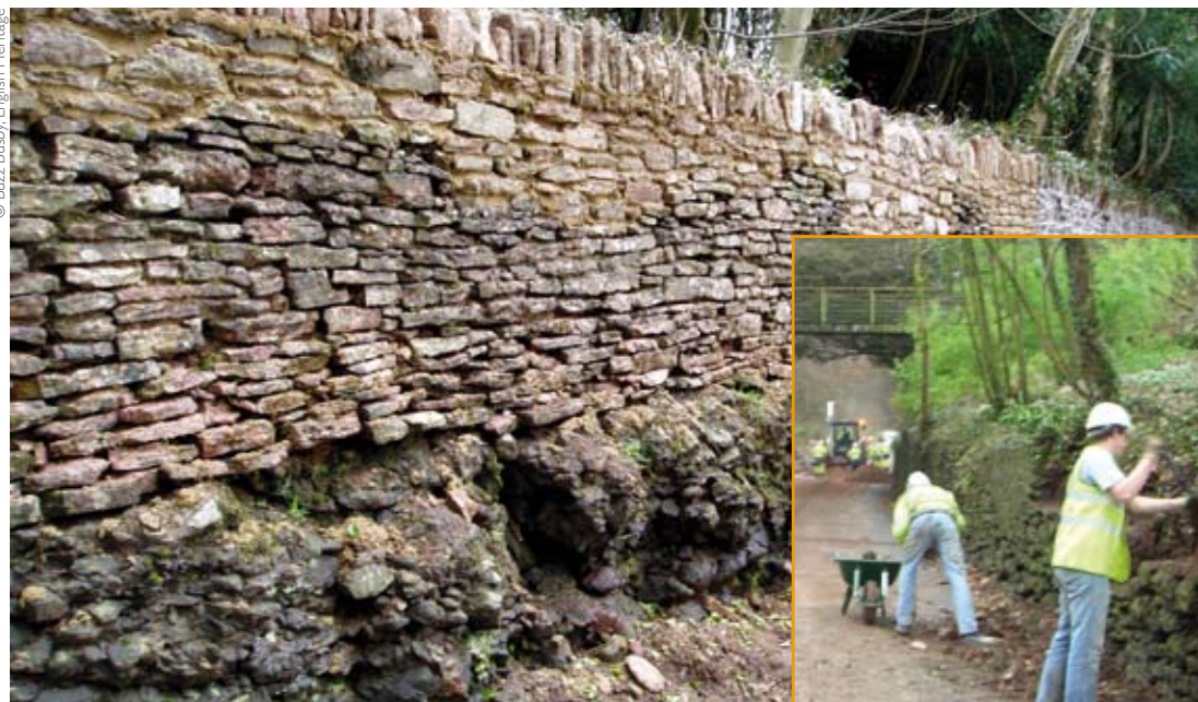
Chewton Mendip Turnpike Wall: Detail of west wall showing deterioration of the living rock foundation of the wall.
