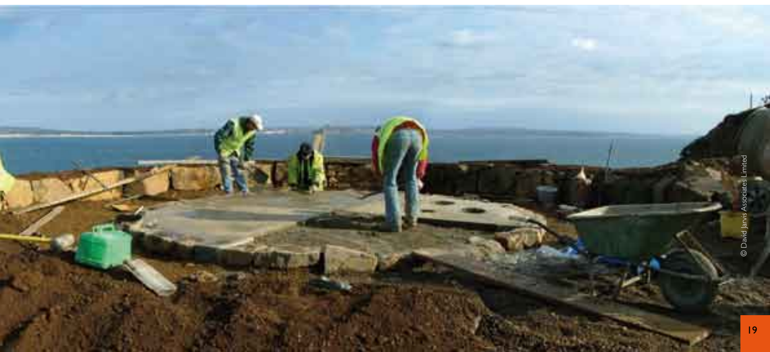
Penlee viewpoint under construction in early 2007
