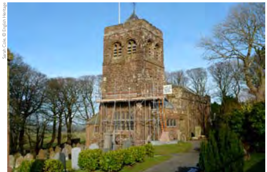
St Michael's Church, Arlecdon during works
