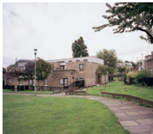
Fig 69 Cluster blocks at Palmerston Walk, Clasper Village. Each block contained four ground-floor flats with four maisonettes above. [AA038439]
