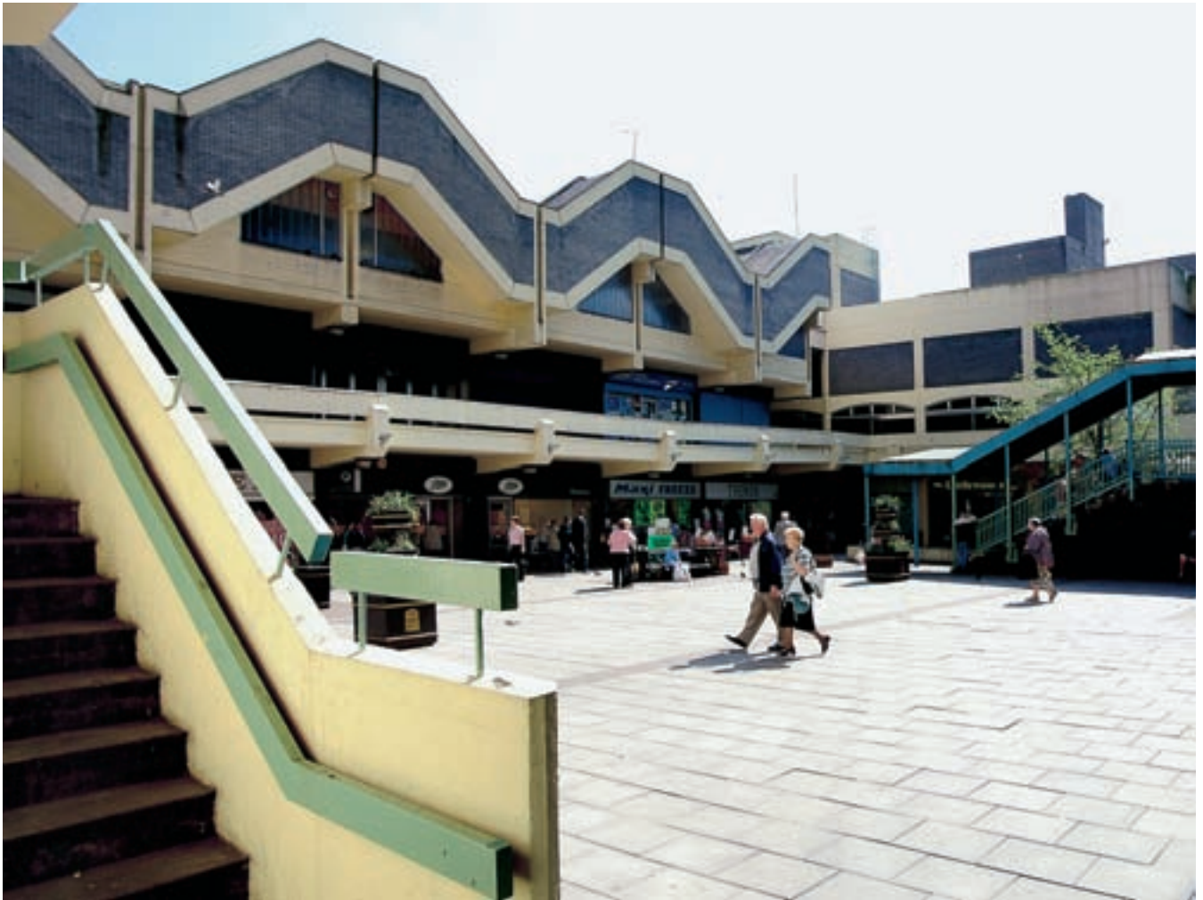
Fig 75 Trinity Square shopping precinct was designed in the mid-1960s and replaced much of Gateshead's old town centre. Very much a period piece, its brutal concrete environments are not sympathetic to 21st-century tastes and many shop units lie empty. [DP000119]
