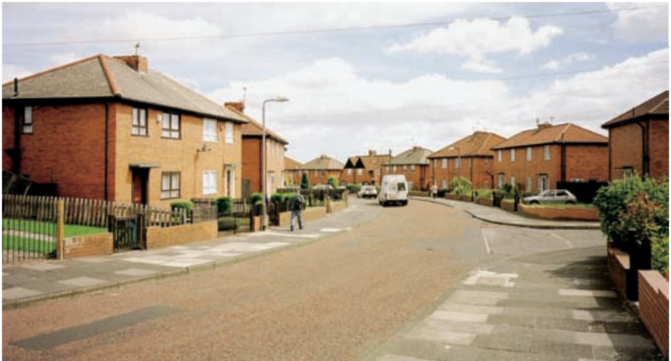
Fig 53 Kingston Road, Deckham Hall Estate, built between 1936 and 1939. The houses on this estate were plainer in appearance than those at Carr Hill or Bensham and were built to a higher density. [AA036521]
