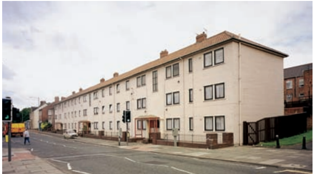
Fig 57 Concrete 'Orlit' flats on Saltwell Road, built between 1952 and 1954 at a time when traditional building materials were in short supply. [AA038431]
