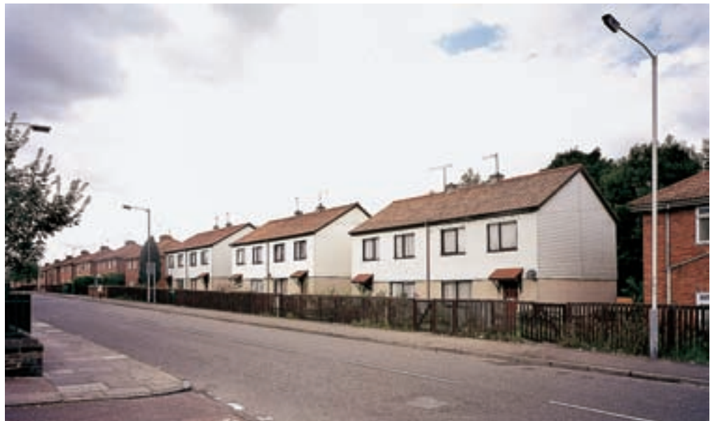
Fig 58 Six semi-detached concrete 'Dorran' houses on Rose Street, built between 1952 and 1954. [AA038436]
