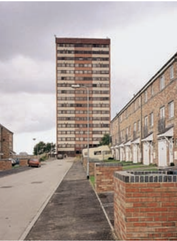
Fig 72 Tyne Views, Windmill Hills, and the earlier St Cuthbert's Court. This development of the late 20th century and the early 21st is on the site of the ill-fated St Cuthbert's Village. [AA038450]
