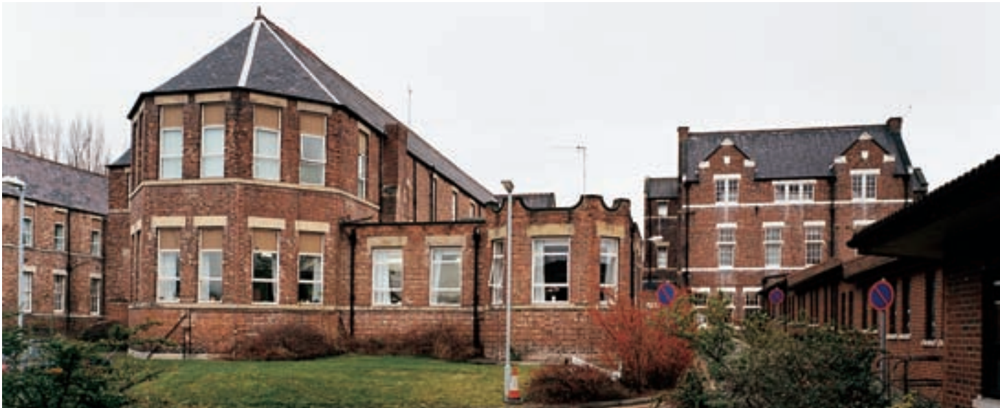
Fig 20 Bensham Hospital was originally built between 1886 and 1890 as the infirmary of Gateshead Union Workhouse. This view shows the central administration block and one of the ward pavilions. [AA040273]
