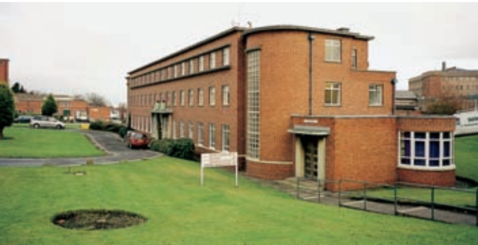
Fig 21 The isolation block at the Queen Elizabeth Hospital, built in the years 1938–40. [AA040361]
