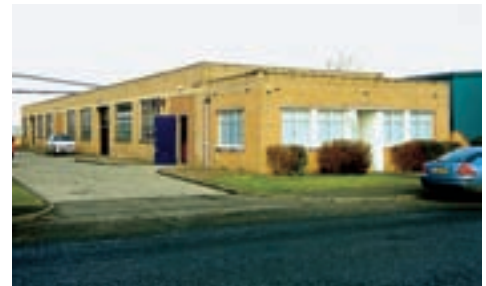
Fig 6 (above, top) A standard factory of 8,000 sq ft (743.2 sq m) on First Avenue. The two-storeyed office block provided a frontage to the factory proper, which was lit from the side walls and by clerestory windows. [DP00043]
