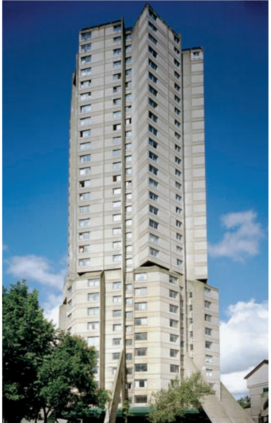
Fig 70 Derwent Tower (196 flats) was designed by Orven Luder and built in 1969. The concrete basin at the bottom was intended to overcome the potential problem of floodwater from the River Team. It is unique in Britain and it is easy to see why it is known locally as 'The Rocket'. [AA038514]
