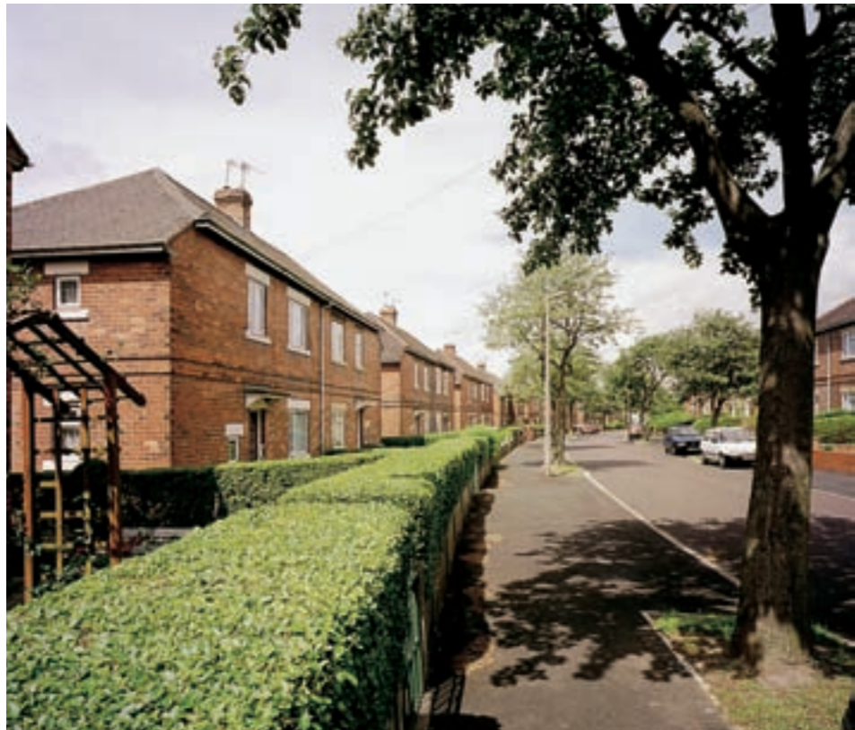
Fig 51 Ascot Crescent, Bensham, built in the mid-1920s. The houses here are similar to those used to extend the Carr Hill Estate. [AA036531]
