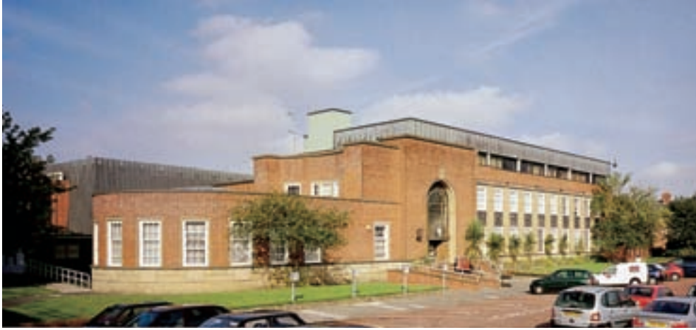
Fig 14 (left) The Borough Treasurer's Department (Civic Centre First Stage), Prince Consort Road, was opened in 1954. The third storey was added between 1972 and 1974 by A Leslie Berry, the Borough Architect. [AA038565]
