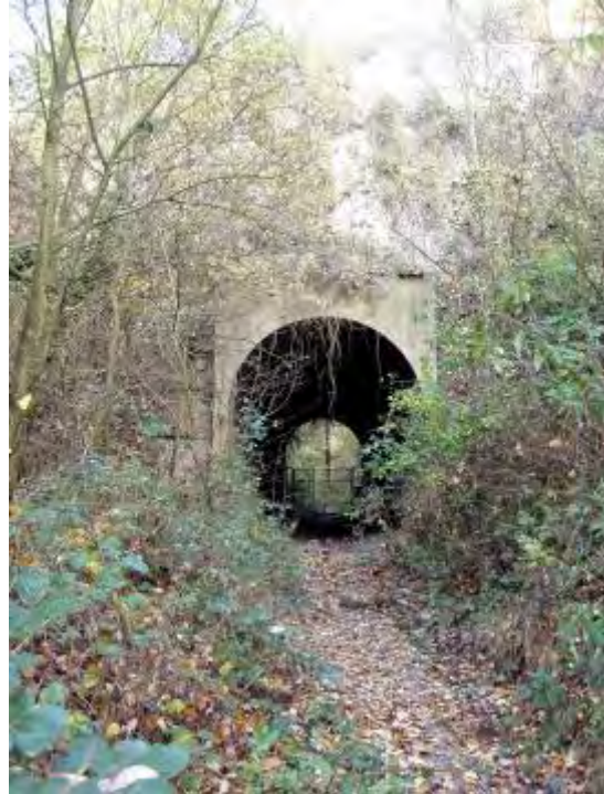
Fig. 28: Crayland Gorge Tunnel, Swanscombe Kent. This tunnel cuts through the chalk spine separating two quarries (photos:ECC/KCC 2004)
