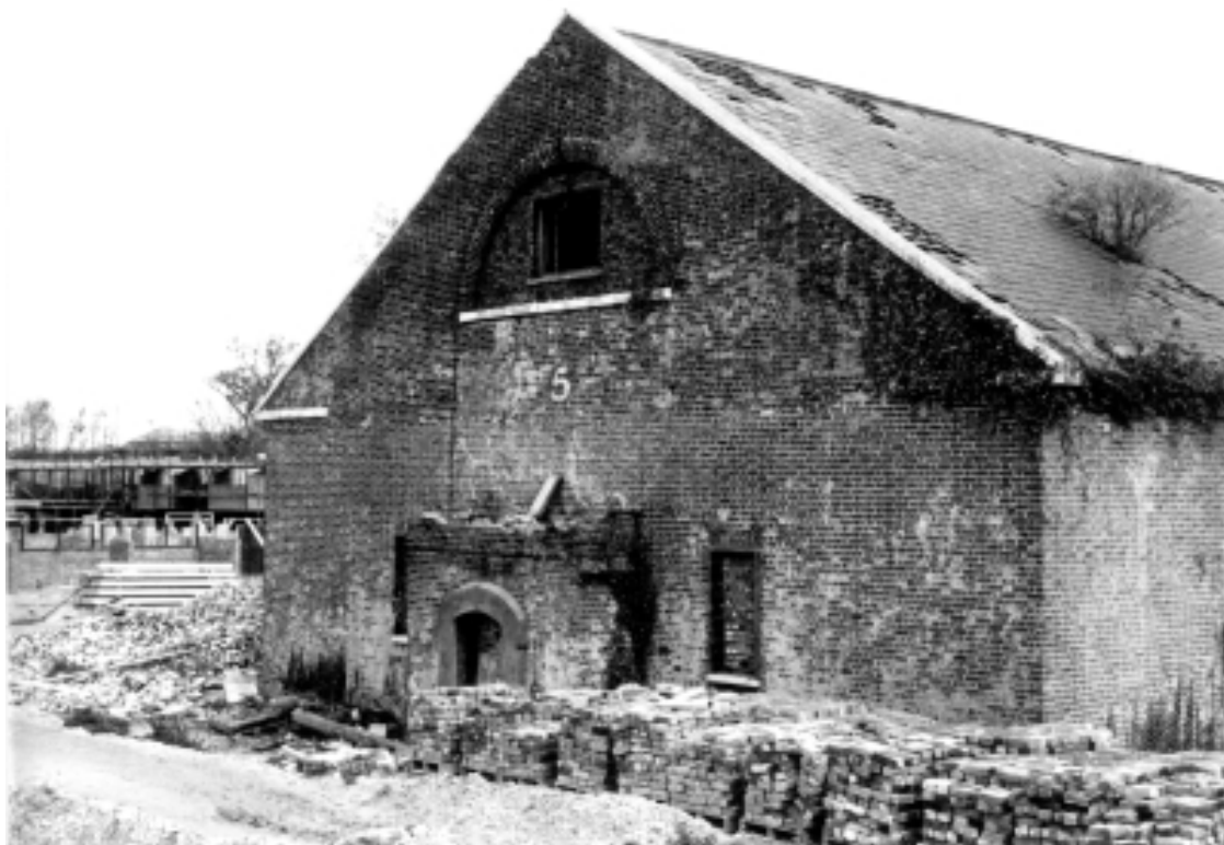
Fig. 30 Magazine No. 5, Purfleet. Constructed by 1765 this magazine would have held up to 9600 barrels of powder. This example is the only survivor of a group which were situated on the north bank of the Thames where the Mardyke enters it.
