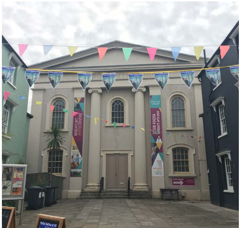
Figure 14: Tregreare Chapel (Grade II) has been converted into residential use. The foreground has been retained as a graveyard and the domestic curtilage keeps around the ancillary accommodation. © Cornwall Council, photographer Tammy White
