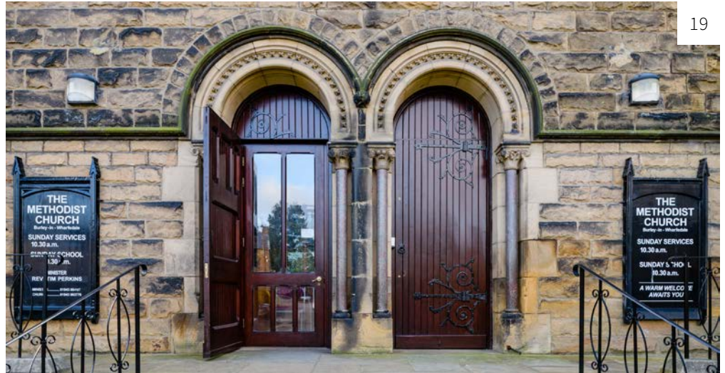
Figure 19: At Burley in Wharfedale Methodist Chapel (Grade II), glazed doors have been installed behind the existing, so that when the church is closed the historic character is retained. © Ian Lamond Photography
