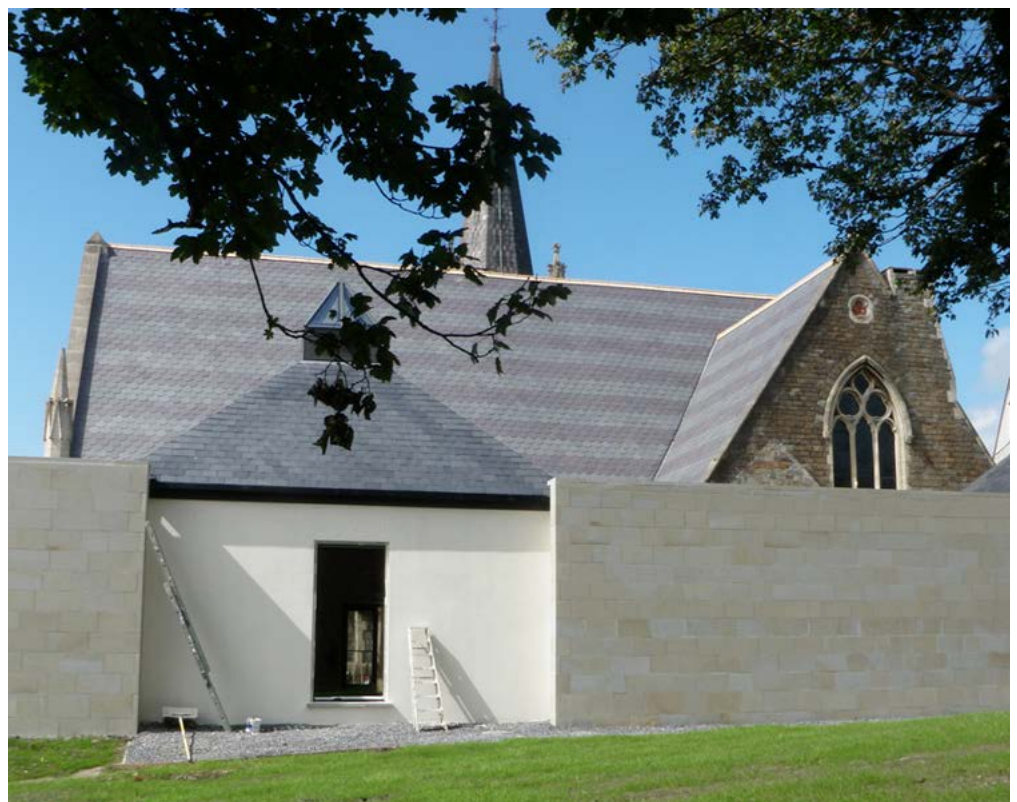
Figures 23 and 24: Four Oaks Methodist Church has mixed contemporary and traditional design to extend the chapel as part of the refurbishment of the hall and to provide additional accommodation. © KKE architects
