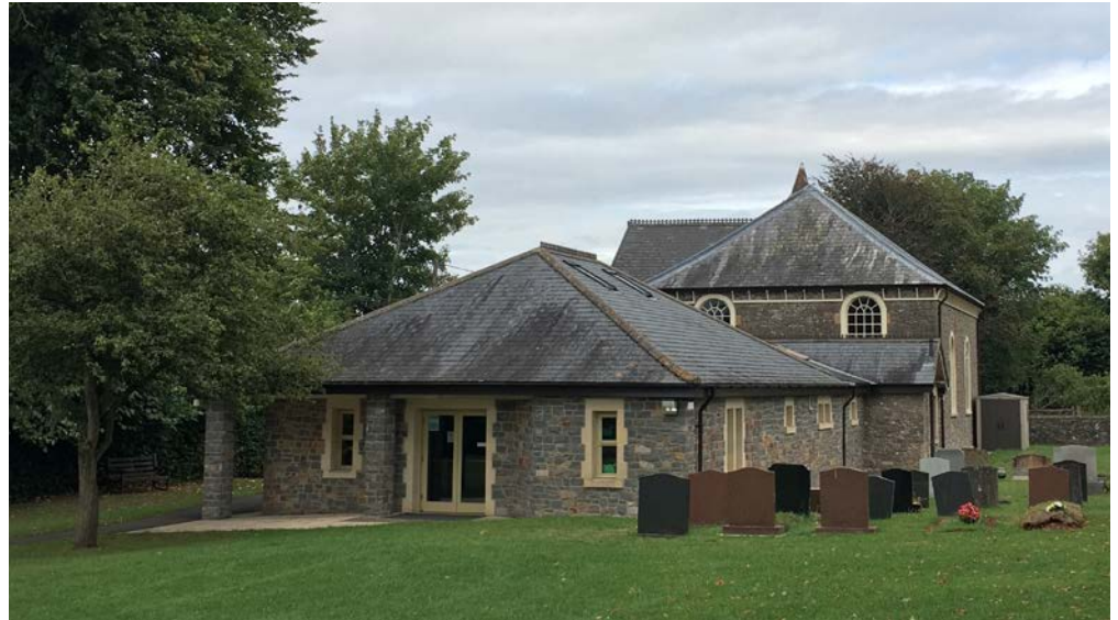
Figure 22: Chew Stoke Chapel (Grade II) was extended with a traditional extension in the 1970s, which continues to respond positively to the overall character of the church.
