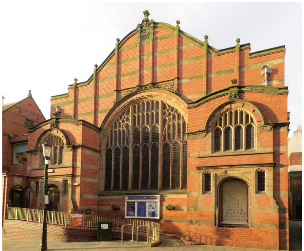
Figure 16: In our experience, it is rare that nothing sympathetic can be done to improve or facilitate access. At the Wesley Centre, Chester, Grade II, an external ramp was created to allow for access into the church. © Wesley Church Centre
