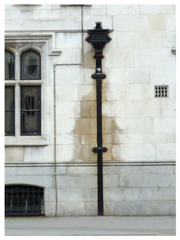
Many damp problems are the result of poorly maintained gutters and downpipes.
