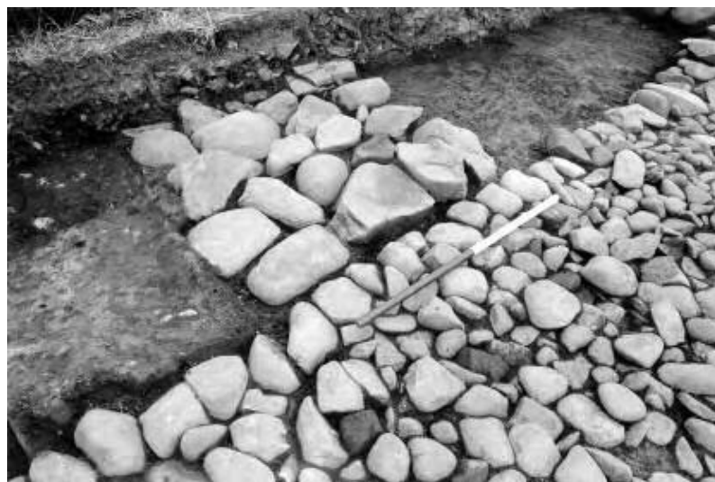
Fig 430 Bowness-on-Solway: foundation for south wall of interval tower.
