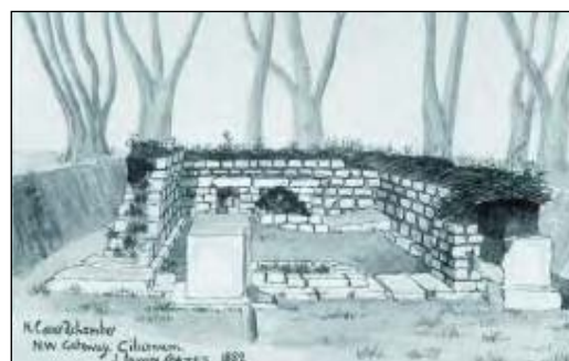
37 N. Guardchamber, N.W. Gateway. Cilurnum. 1882 (Fig 45) The sketch, looking north, shows the internal view of the guardroom, including the pivot block and slot for the gate. At the north end is a stone water channel and a stone platform to support a tank for the water supply. The west wall of the guard chamber is seven courses above the offset course. The guard chamber door threshold is in place. A clump of mature trees, north of the chamber, extends across the Ditch and fort wall.
