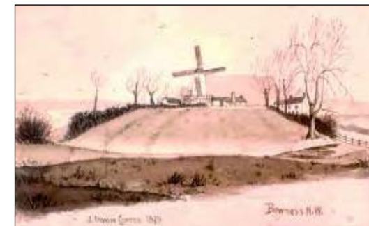
165 Bowness N.W. 1879 (Fig 172) The depiction shows a windmill with four sails or 'sweeps' and wooden cantilevered gantry situated in the north-west corner of the fort together with the kiln and associated buildings (Hughes 1973, 355). The windmill, owned by Sarah Lawson, was demolished between 1880–85 (Hughes 1972, 126). A section of the water-filled west Ditch of the fort is outlined. Ridge and furrow are evident in the field in the north-west corner of the fort. Mill Cottages are seen on the south side of the Bowness-Silloth road.
