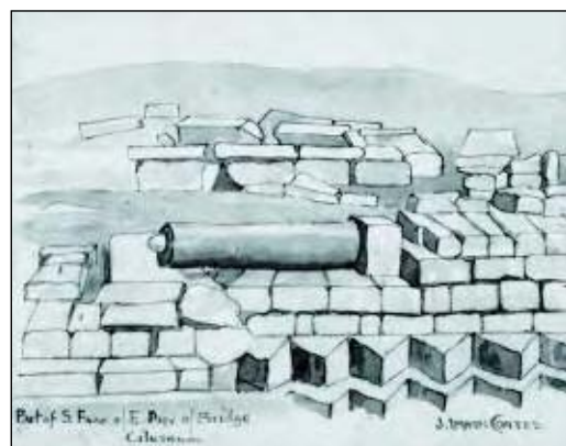
35 Part of S. Face of E. Pier of Bridge. Cilurnum. no date (Fig 43) Presumably made at the same time as Figs 41 and 42, the sketch depicts a cylindrical column, with an oval boss at one end and a square base at the other, lying on the masonry of bridge two. The lower blocks of the abutment have been laid at an angle of 45 degrees to those above to form a series of dogtooth courses. A number of blocks forming the stone millrace are in the background.
