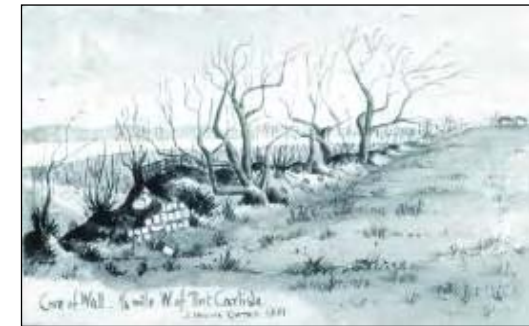
164 Core of Wall ~ 1/4 mile W. of Port Carlisle. 1881 (Fig 171) The site is west of Mc79. The view, looking east, shows the line of the Wall although it is covered in trees and bushes and a wooden fence has been erected on top. Three courses of the south face of the Wall are visible at the west end but much has been robbed (Jenkinson 1875, 187). In the background several houses in Port Carlisle are depicted.
