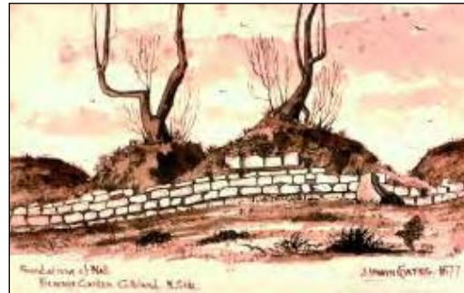
131 Foundations of Wall. Vicarage Garden. Gilsland. N. Side. 1877 (Fig 138) Up to five courses of Wall face are visible, the top of the Wall being covered in turf with two trees growing from the mound. Three cuttings have been made across the width of the Wall and in front are four small piles of Wall core. This section of Wall had been exposed not long prior to this by the vicar of Gilsland, Rev A Wright (Ferguson 1877-8, 24).
