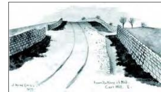
23 Foundations of Wall, Carr Hill, E. 1879 (Fig 31) The line of the north face of the Wall is visible in the road surface. A stone boundary wall, probably incorporating Roman material, runs parallel to Hadrian's Wall and to the road. The slope of the north Ditch is discernable. The view is close to the position of T20a.
