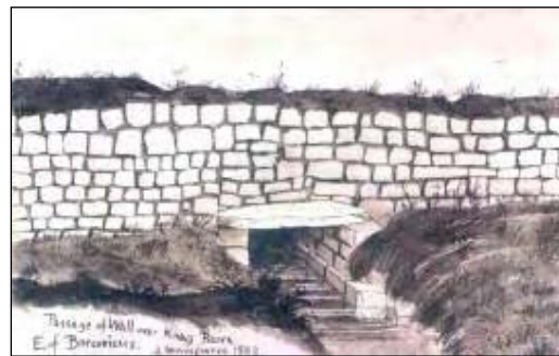
88 Passage of Wall over Knag Burn E. of Borcovicus. 1882 (Fig 96) A detail of the south face of the Knag Burn culvert with eight courses of Wall visible. A large stone slab covers the culvert, the east side of which has three courses of large blocks above an offset course. The top of the Wall is turf-covered.
