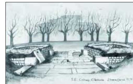
40 S.E. Gateway. Cilurnum. 1879 (Fig 48) The first gate to have been excavated, perhaps in 1854, but before 1863 (Bidwell and Snape 1993, 13); the sketch shows the two guard chambers and the paving slabs of the single passage portal in the east wall. The outer face of the fort wall is partially excavated. The north pivot block is in place and a large block with a pivot hole rests against the north wall of the south guard chamber. Irwin Coates clearly depicts guard chambers on either side of the gate. These are not evident on the ground or indicated on any of the site plans, and no doors are visible in the side walls of the portal, the entrance perhaps being at the back of the guardrooms. Mature trees are growing within the fort.
