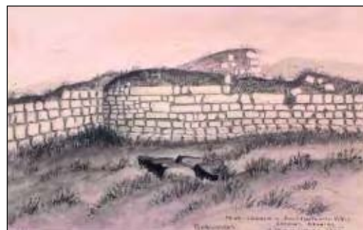
80 N.W. Corner & Junction with Wall showing repairs, Borcovicus. 1883 (Fig 88) Five courses of the south face of Hadrian's Wall are depicted at the north-west corner of Housesteads fort. The fort wall itself is built on top of the offset course. A number of large blocks in the external face of the north wall of the fort indicate Roman repairs. Within the fort some of the west wall of the north-west angle tower is visible. Both the fort wall and the Curtain Wall are turf capped. Three large pieces of masonry lay outside the fort.
