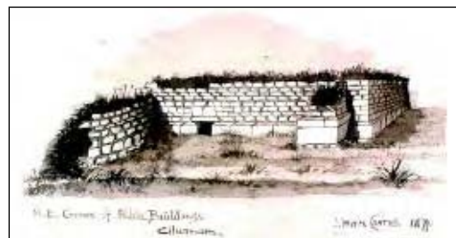
78 N.E. Corner of Public Buildings, Cilurnum. 1877 (Fig 86) The drawing is of the north-east corner of the Commanding Officer's House showing the moulded plinth, the buttress and the curve of the apse end of the bathhouse. The east wall has an outlet at plinth course level. The walls survive up to eight courses above the plinth.
