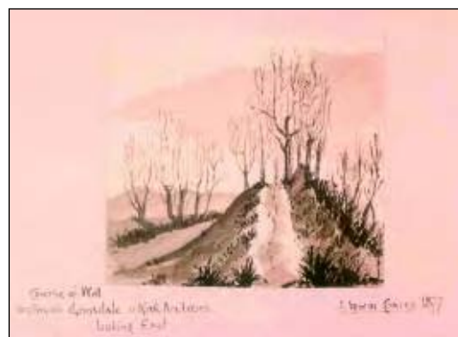
146 Course of Wall between Grinsdale & Kirk Andrews, looking East. 1877 (Fig 153) The depiction is of Long Bank between Ladylands Lane and Kirkandrews. The earth-covered mound of the Wall has a hedgerow growing on top as well as a group of mature trees. A footpath is on the berm with the ground sloping away to the north Ditch.
