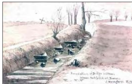
162 Foundations of Bridge in Stream between Port Carlisle and Bowness. 1879 (Fig 169) The depiction shows three large wedge-shaped blocks, which must have been associated with a Roman culvert through the Wall, partly exposed in the bank of a watercourse, which flows in a northerly direction into the Solway Firth. The Wall crosses the stream close to the estimated position of T79a. The nearest block seems to have a recessed hole in the top. A number of blocks and stones are in the bottom of the stream. A small sketch gives the measurements between the blocks: 3ft (0.9m) between the north and central blocks and 6ft (1.8m) between the central and southern blocks. The sketch shows a similar shaped block in the east bank of the stream. No discernable traces of the Wall or Ditch remain but a path or track follows the line of the stream and this indicates the line of the Wall. In the distance are the roofs of two buildings and a four-sailed windmill in Bowness village.
