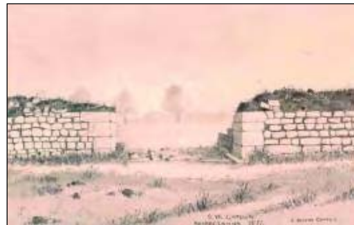
133 S.W. Gateway. Amboglanna. 1877 (Fig 140) This single portal gate had been exposed in 1850 (Birley 1961, 199) The drawing, from the west, shows the pier blocks on both sides of the gateway with up to eight courses of facing stones in place as well as the portal threshold within which are blocks of fallen masonry. The top of the fort wall is turf covered. Several mature trees are depicted inside of the fort.
