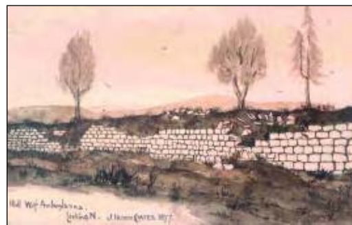
140 Wall W. of Amboglanna. Looking N. 1877 (Fig 147) The south face of the Wall west of Birdoswald stands at least seven courses high, the earth capping containing core work. Sections of the Wall face show evidence of either collapse or robbing of the stone work. Three mature trees are shown on the north side of the Wall. In the distance to the north-west is the outline of the only remaining wall of Triermain Castle, which had been built with re-used Roman Wall stone.
