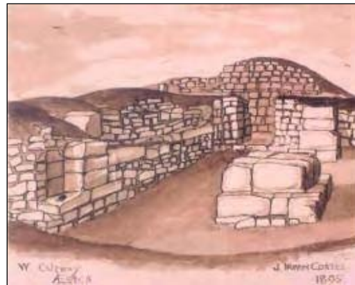
115 W. Gateway. Æsica. 1885 (Fig 123) The internal view from the south-east shows the blocking in the north portal of the west gate, the spina blocks and the north guard chamber with its doorway (seven courses high), all of which had been uncovered in June of that year by J P Gibson (1903, 26). Within the blocking of the north portal are the two pivot blocks for a later raised Roman road surface. The north pivot block of the south portal is in place including three of the pier blocks above the portal blocking. In the internal north wall of the guard chamber there are five courses below the string course and five courses above. The gateway blocking and the walls of the guard chambers are turf-covered.
