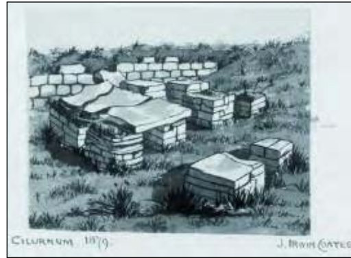
43 Cilurnum. 1879 (Fig 51) The drawing depicts a section of the hypocaust system within the central part of the Commander's House. Three large stone slabs rest upon raised stone pillars with another slab in the background resting against five courses of walling.
