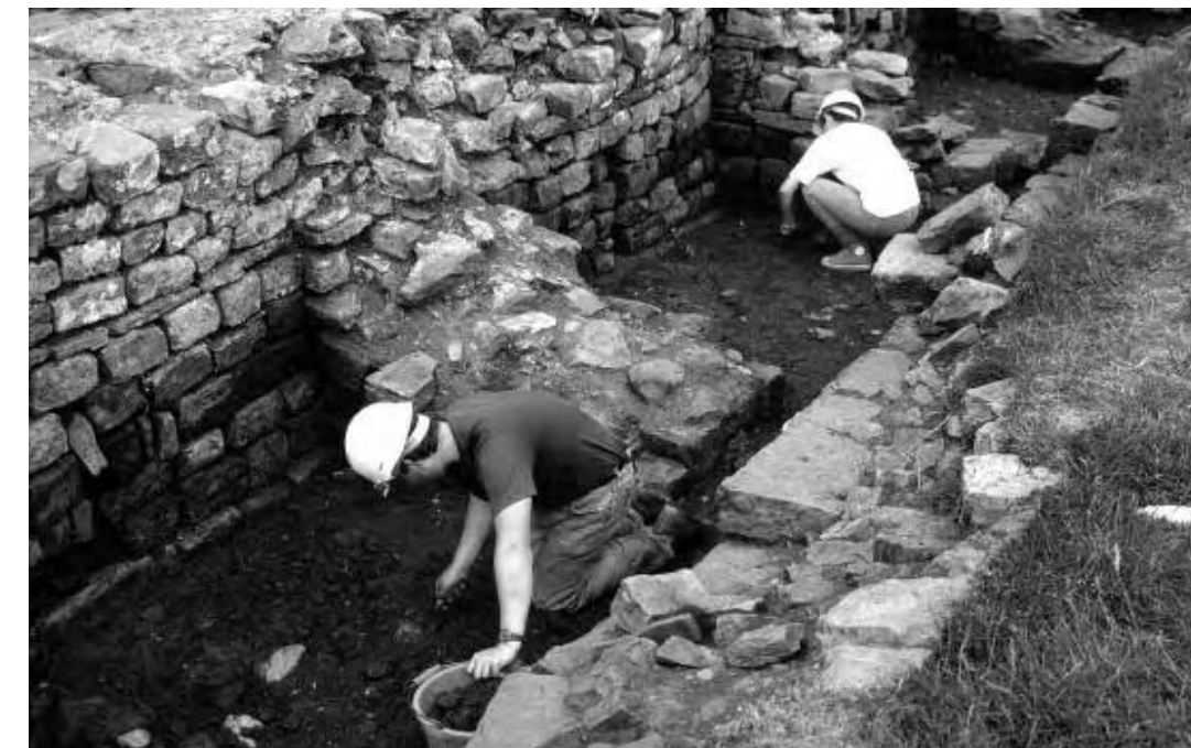
Fig 5 Excavation in progress on the south horreum at Birdoswald in the first season in 1987.
