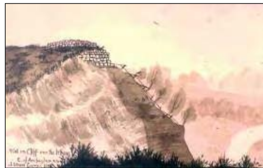
132 Wall on Cliff over the Irthing E. of Amboglanna. 1879 (Fig 139) This shows the section of Wall east of Mc49 (Harrow's Scar) overlooking the steep west bank of the Irthing river. At least nine courses of facing stones are visible above two courses of foundations, the rest of the Wall having been taken away by land slips. The bare slope above the curve of the river has a wooden fence and a line of five trees. An 1848 watercolour by H B Richardson (Bidwell 1989, pl 6) shows the Wall perched on top of the river escarpment and evidence of the river undermining the Wall.
