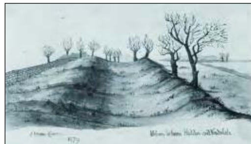
18 Vallum between Heddon and Vindobala. 1879 (Fig 26) The view, looking east, shows the slope of the Vallum Ditch and its two mounds. A stone boundary wall north of the Vallum, probably containing re-used Roman stone, is situated on the south side of the Military road. The depiction is in Wall-mile 12, probably close to T12b.
