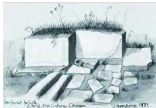
38 Iron Socket for Gate. S. Portal. N.W. Gateway. Cilurnum. 1882 (Fig 46) This shows a detail of the surviving iron collar in the pivot block to hold the door as well as the south portal threshold block.
