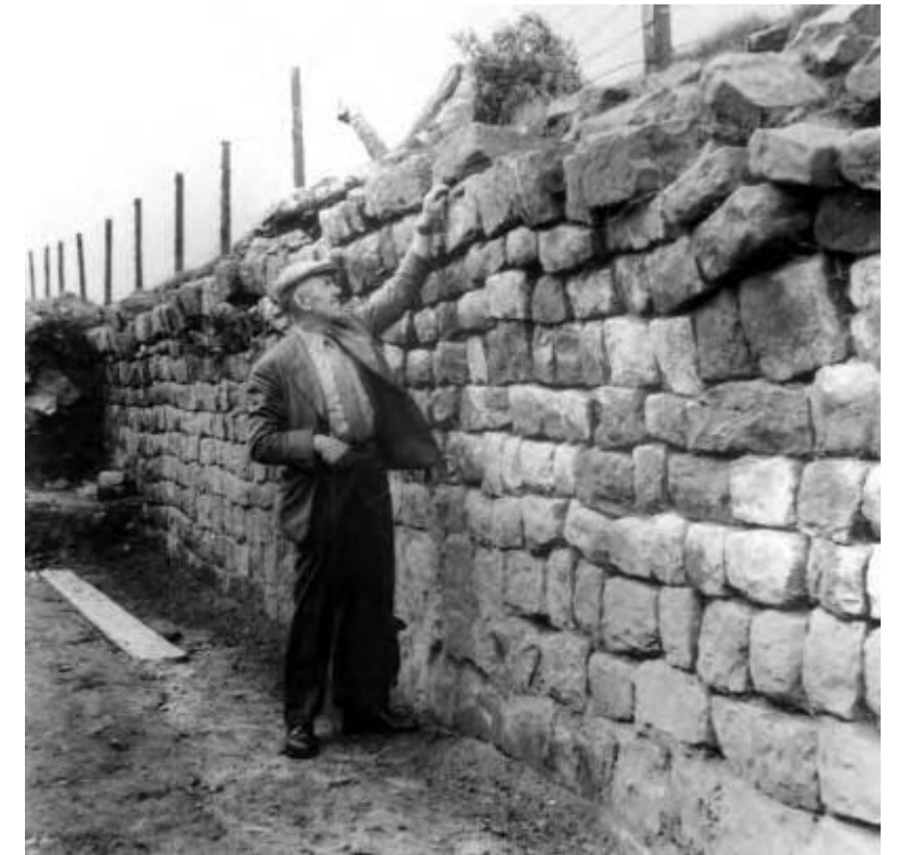
Fig 174 Charles Anderson inspects the Wall east of Birdoswald.
