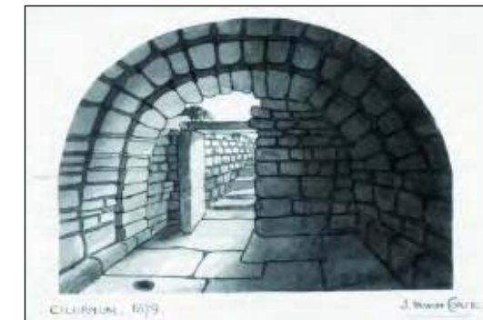
50 Cilurnum. 1879 (Fig 58) The internal view of the underground strong room in the principia shows the arch-ribbed vaulting and entrance with its monolithic door jam and a stone slab over the passage steps. The walls of the vault are built on a stone plinth. On one of the floor slabs is what appears to be a circular drain hole.
