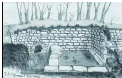
46 Part of Hypocaust. Cilurnum. 1882 (Fig 54) This is the east wall of the Commanding Officer's House at the south-east corner showing the brick arch of the furnace through the wall. A string course extends the length of the east wall. Large foundation blocks and the north wall of eight courses (above a moulded plinth) of a small room abut the east wall. The top of the east wall is turf capped and a clump of a dozen mature trees is situated within the fort.
