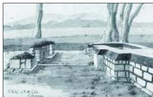
36 S. Portal of N.W. Gate. Cilurnum. 1882 (Fig 44) The view, from the west, shows the south portal, gate threshold and central spina of the West gate. Hadrian's Wall is bonded with the south guard chamber, which stands three courses above the offset course. Several mature trees grow adjacent to the gate.
