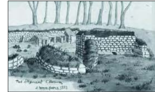
47 Part of Hypocaust Cilurnum. 1882 (Fig 55) The view shows the raised floor and hypocaust of the Commanding Officer's House together with the apsidal ends of the hot room and the moulded base course on the external face of the east wall. A squared-topped column rests against the wall close to the hypocaust. All of the walls are turf capped. A clump of eleven mature trees is depicted within the fort.
