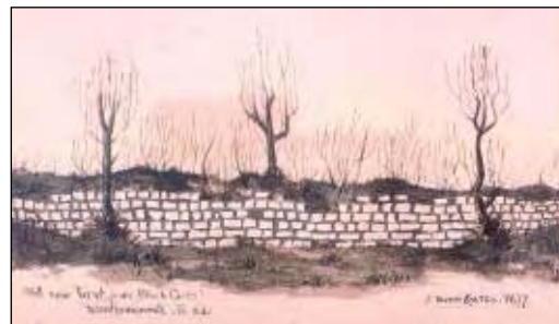
71 Wall near Turret (near Black Carts) recently uncovered – S. side. 1877 (Fig 79) Excavated in 1873 by Clayton, the Wall stands at least six courses high. Vegetation and trees are on top of and adjacent to the Wall.
