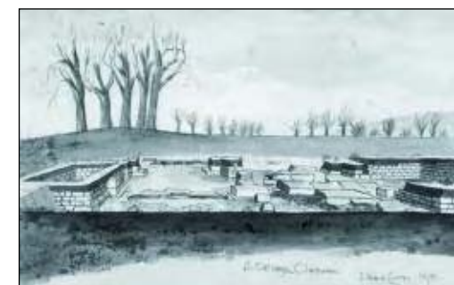
39 S. Gateway. Cilurnum. 1879 (Fig 47) The drawing, looking north, shows the east and west guard chambers, central spina and gate portals. The sill and threshold of the east portal have been uncovered, while the east portal retains the large blocks of a later road. Within the fort are a large number of mature trees.
