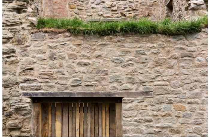
Country Landscapes Partnership. The works included rebuilding part of one demolished wall to ensure structural stability, stone renewal, repointing and soft capping of exposed wall heads. The works were concluded in April 2017 and the structure removed from the Heritage at Risk Register.
