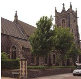
© Nicholas Warns Architects
