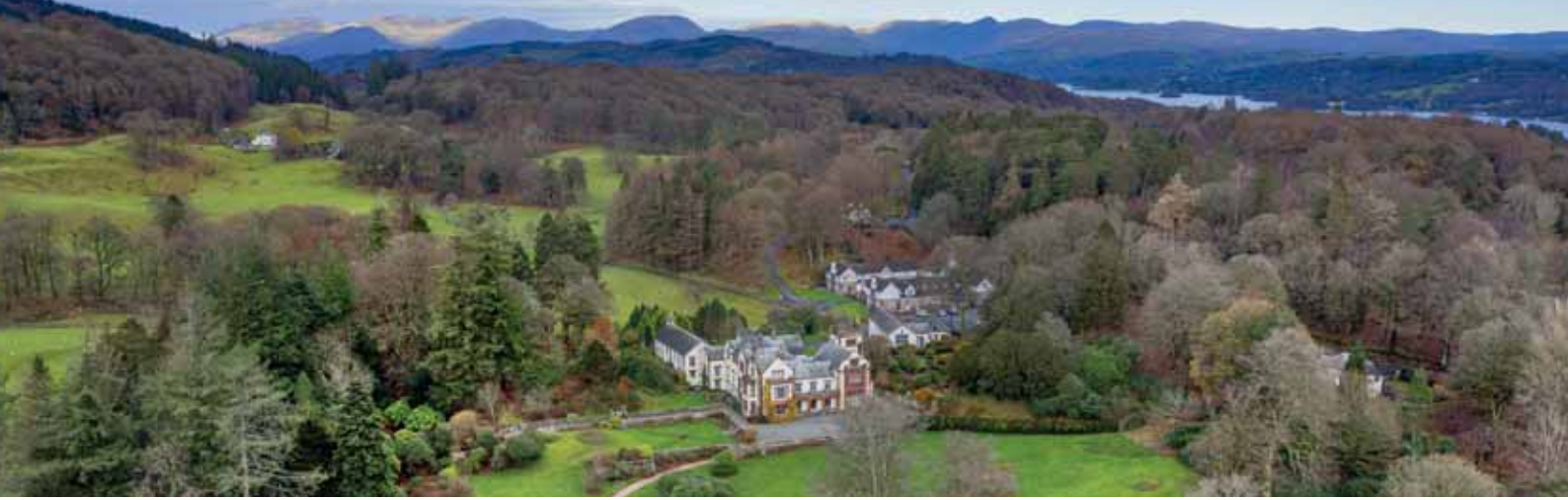
Grade II* listed gardens at Graythwaite Hall, Ulverston, Cumbria
