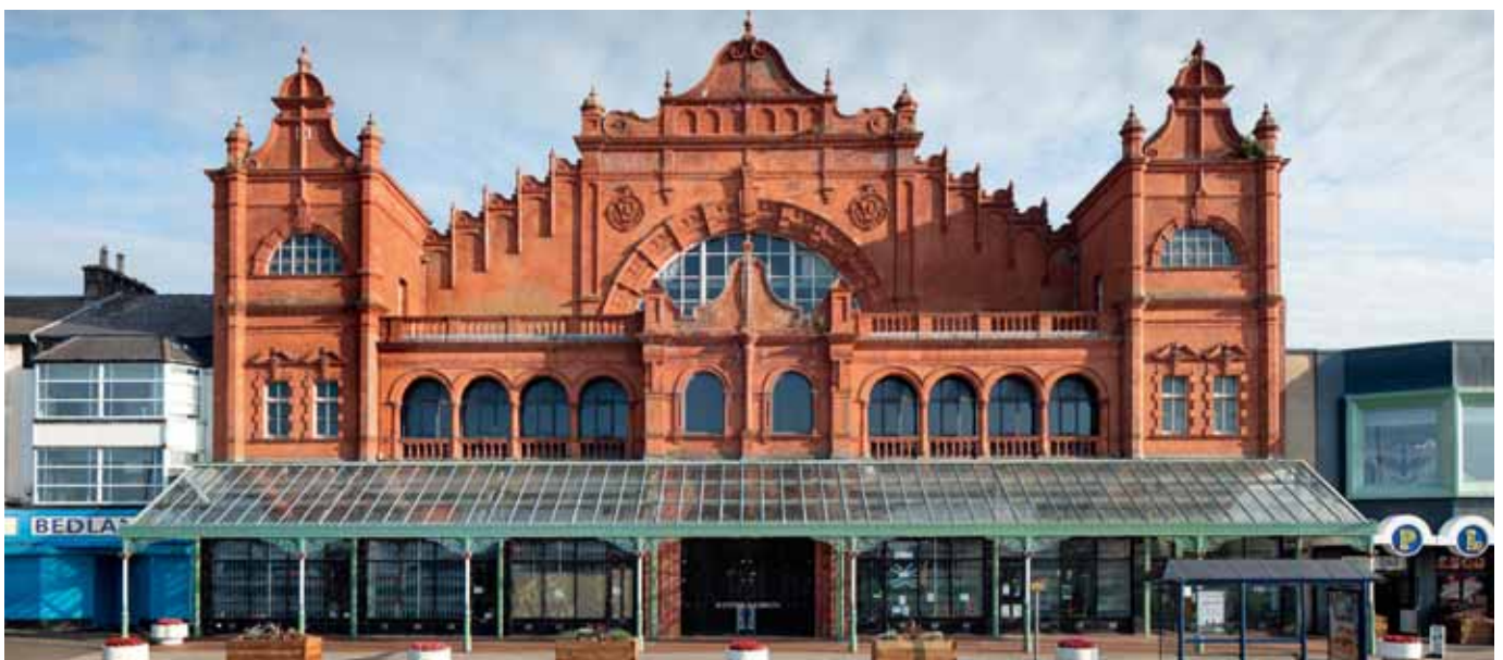
Morecambe Winter Gardens, Lancashire. A Heritage at Risk property that benefitted from the Culture Recovery Fund
