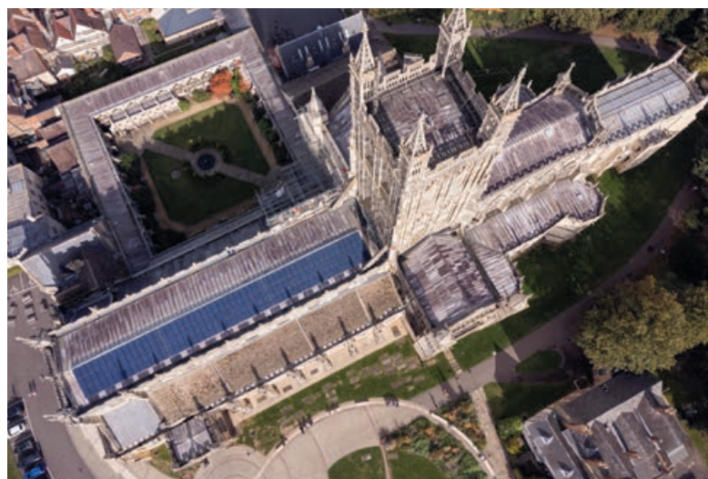
Solar panels fitted on the roof of Gloucester Cathedral
