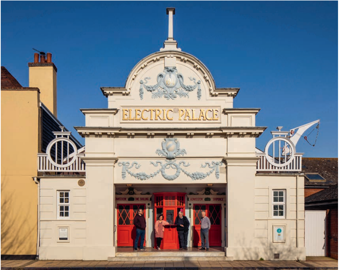
The Electric Palace Cinema, Harwich, following restoration works partly funded by the Cultural Recovery Fund
