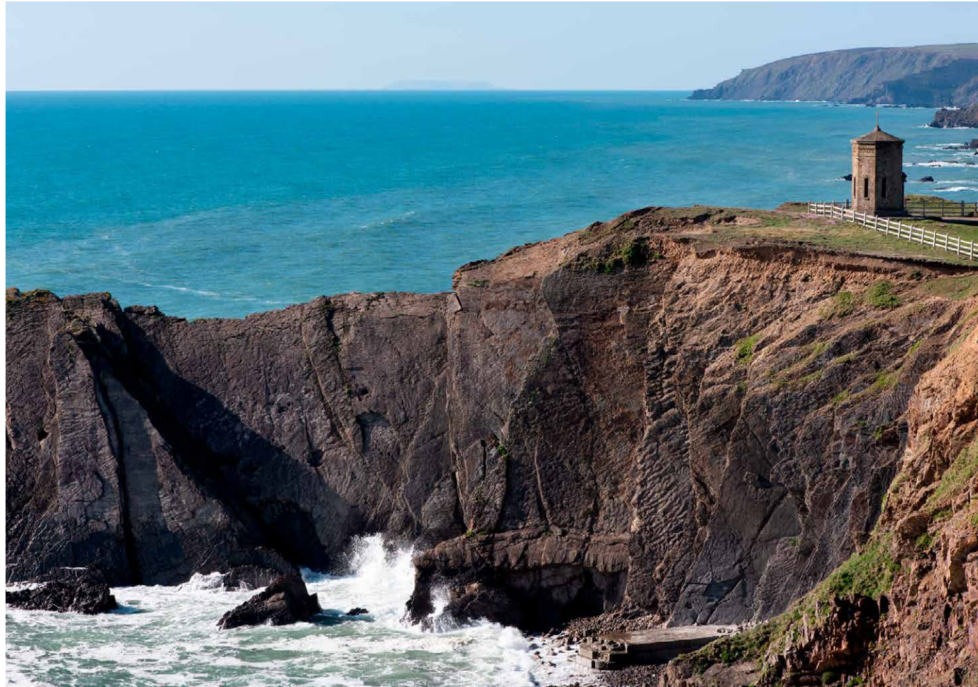
Above left: Bude Storm Tower, Cornwall – adaptation due to coastal erosion. The relocation of a Grade II listed coastal look-out and eye catcher is planned, due to coastal erosion and associated threat of collapse into the sea. © Historic England Archive. Photographer James O Davies, DP276200
