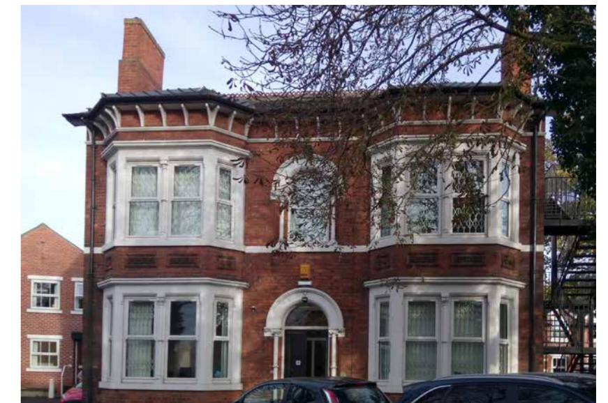
Right: Rosebery House, built for George Pearson, bleachworks owner, in 1884. © Claire Price
