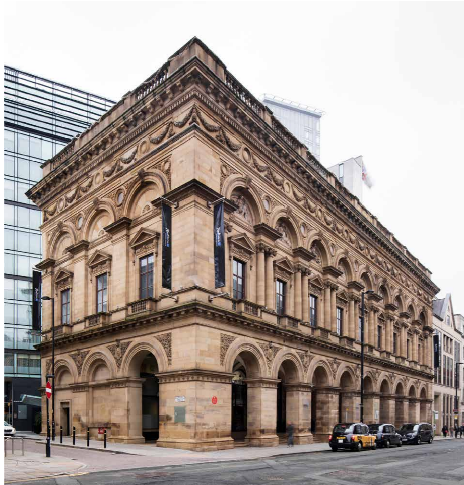
Left: The Free Trade Hall, Manchester, which saw the first acts of militancy by Christabel Pankhurst and Annie Kenney in 1905. DP220475 © Historic England
