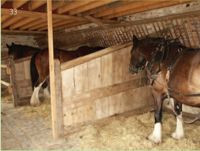
33 A typical stable interior for working horses, showing the stalls that prevented the horses biting and kicking each other; the hay rack and cobbled floor: (Dorset Downs and Cranborne Chase) © Bob Edwards
