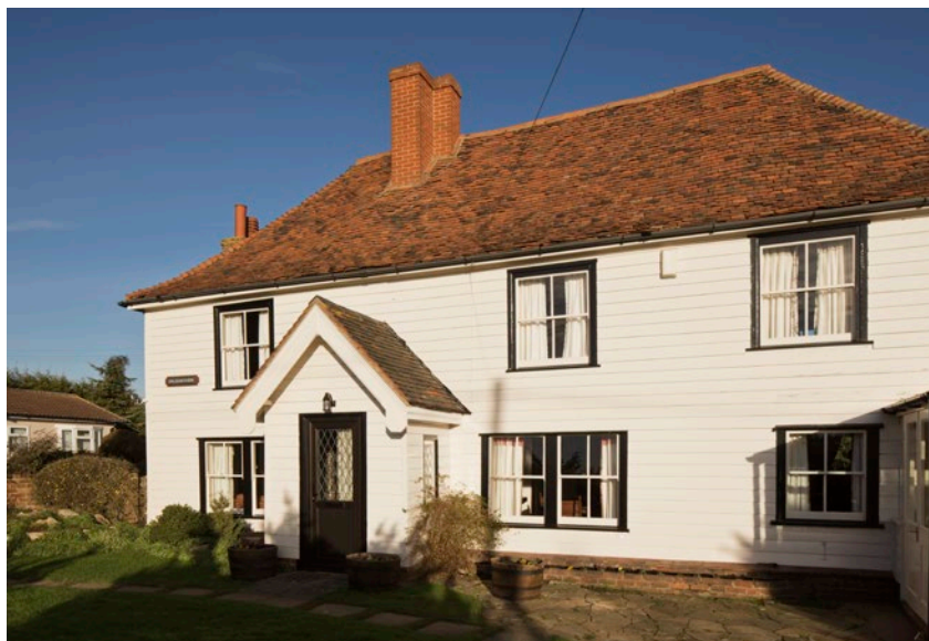
Figure 64 Weatherboarding, such as seen here on the late 16th-century Grade II listed Great Dalham farmhouse in High Halstow, was added to buildings on the peninsula from the late 17th century to protect timber frames. [DP172146]
