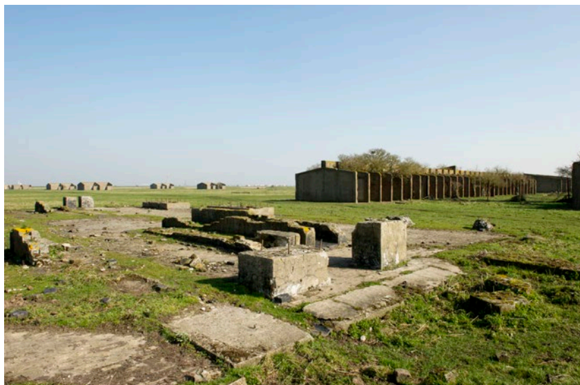
Figure 28 HM Cordite Factory formed part of the extensive explosives works of Curtis's and Harvey Ltd. This photograph shows the remains of the acetone recovery buildings in the foreground and extending off to the right, with cordite blending houses in the distance on the left. [DP141667]
