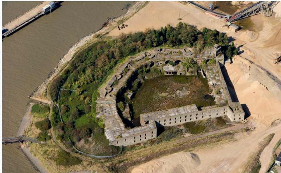
Figure 42 Built in the 1860s, Cliffe Fort was one of three forts constructed where the Thames turns northwards downriver of Tilbury and Gravesend. An arc of granite-faced casemates fronted the river, with barracks to the rear. It remained in use as a battery until the 1920s and served as a base for the Royal Navy Auxiliary Service during the Second World War. 30 [26474/020]
