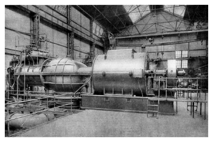
One of the enormous turbo-generators at Carville 'A', Wallsend. Manufactured by CA Parsons, of Newcastle, their normal capacity of 700 electrical horsepower
