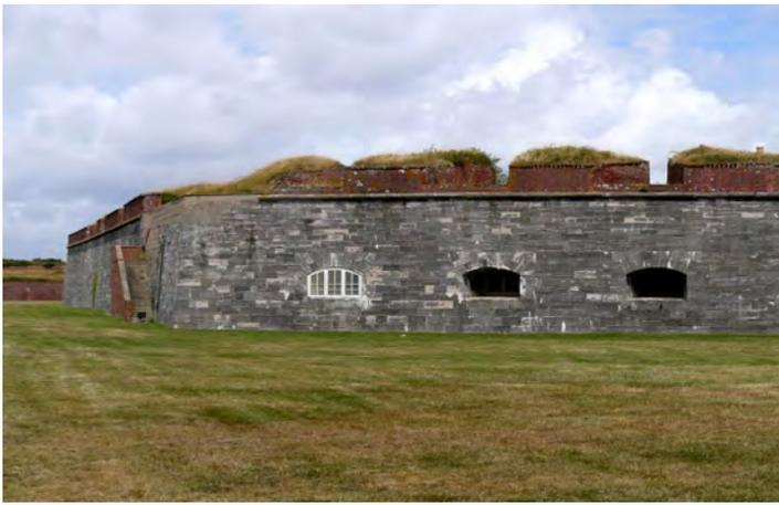
Fig. 6. Fort Cumberland, Hampshire, 1795-1812, was the last fully bastioned fort to be built in England. This picture shows one of the bastions with casemates, in which guns were placed to defend the ditch and adjacent wall.
