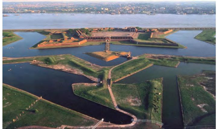
Fig. 5. Tilbury Fort, Essex, designed by the Dutch engineer Bernard de Gomme and completed in 1684 is one of the finest examples of an angled bastion fortification in England.
