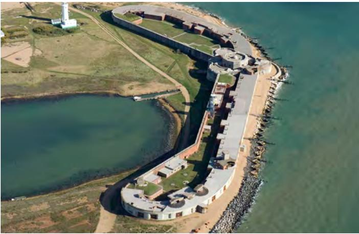
Fig. 8. Hurst Castle, Hampshire. In the 1860s, to protect the western entrance to the Solent and Portsmouth dockyard Henry VIII's fort was encased by two granite faced wing batteries, its guns housed in casemates with iron shields.
