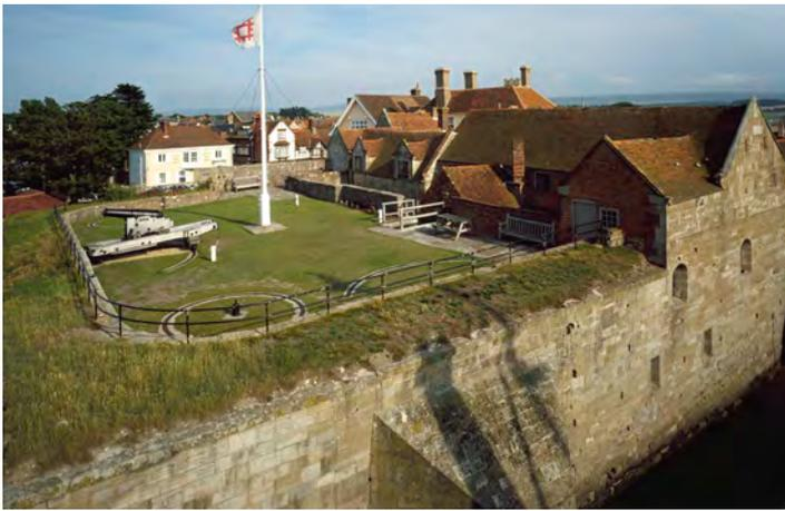
Fig. 2. Yarmouth Castle, Isle of Wight. Elements of this castle represent one of the earliest examples of angle bastion defence in England. The interior was filled in the 1560s to create a large gun platform.
