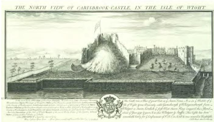
Fig. 4. Carisbrooke Castle, Isle of Wight. A Samuel and Nathaniel Buck print of 1733, showing part of the new bastioned defences erected between 1597 and 1601 to protect the island against possible Spanish attack.
