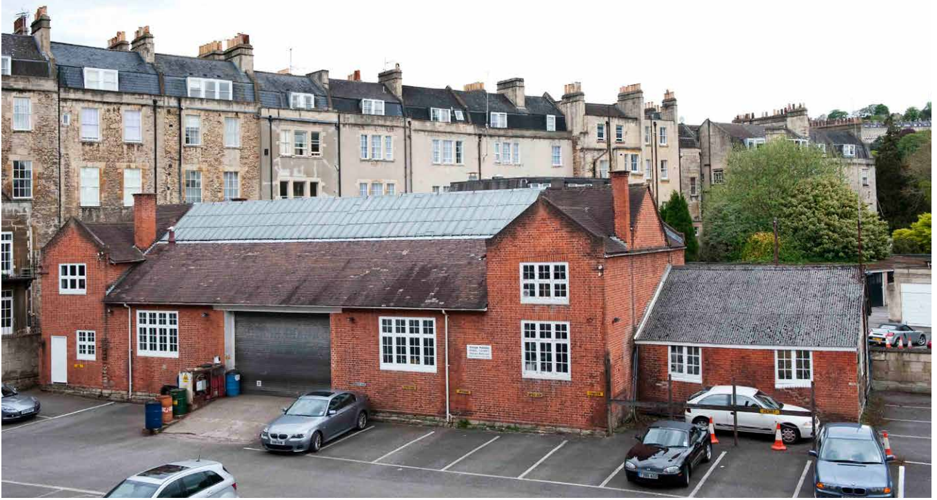
Figure 12 A small number of parking garages built for hotels prior to the First World War are still in use as garages: this, of 1907, served the Pulteney Hotel in Bath.
