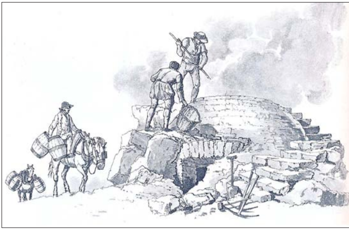
Fig. 4. Lime burners at work firing a flare kiln (1804).
