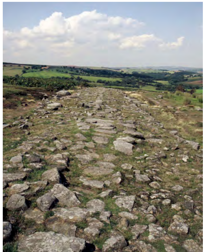
Figure 7 A mile-long stretch of a probable Roman road crosses isolated moorland at Wheeldale, North Yorkshire. Its hardcore and drainage ditches can be seen.
