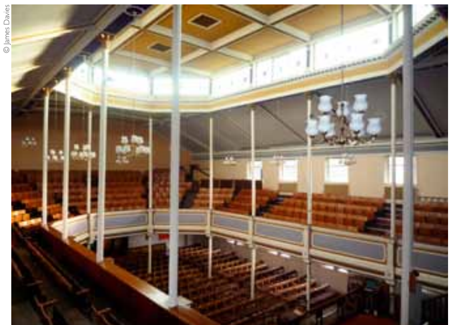
Interior of Methodist Central Hall, Longton, Staffordshire (1841-42)
