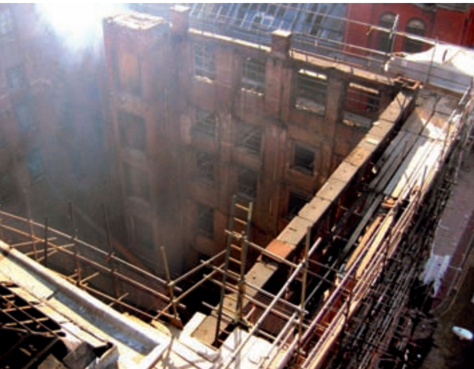
Fig 2 The burnt-out shell of a warehouse in Dale Street. The scaffolding had been erected for the refurbishment that was underway in May 2007 when the accidental fire occurred. [Courtesy of Manchester City Council]
