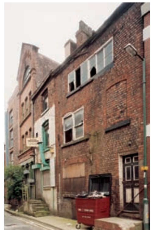
Fig 9 (below) 36 Back Turner Street before it collapsed in 2005. Note the header-bond brickwork and the original three-window arrangement on the first floor. [AA006123]
