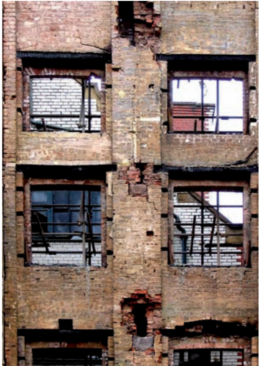
Fig 3 The fire-ravaged internal walls of a warehouse in Dale Street. Note the charred wooden lintels to the windows and broken brick work where metal floor-beams have collapsed under the intense heat. [Courtesy of Manchester City Council]
