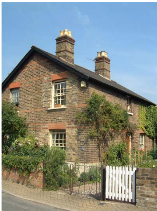
Alexandra Cottages: Sash windows reinstated in restored openings
