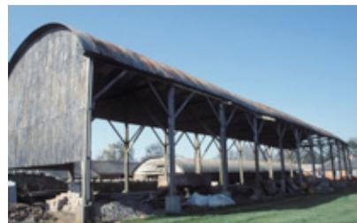
Dutch barns were first built of timber and corrugated iron, and then a mixture of timber, iron and steel frames. They became standardised from the 1880s when firms began to advertise and issue printed details with drawings, usually along with other 'kit buildings' such as parish halls. Photo © Joan Grundy
