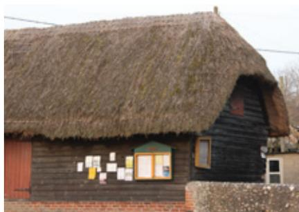
Longstraw is distinguished by its much thicker and looser covering of straw. The ears and butts are mixed, and the stems are bruised and crushed. Photo © Bob Edwards
