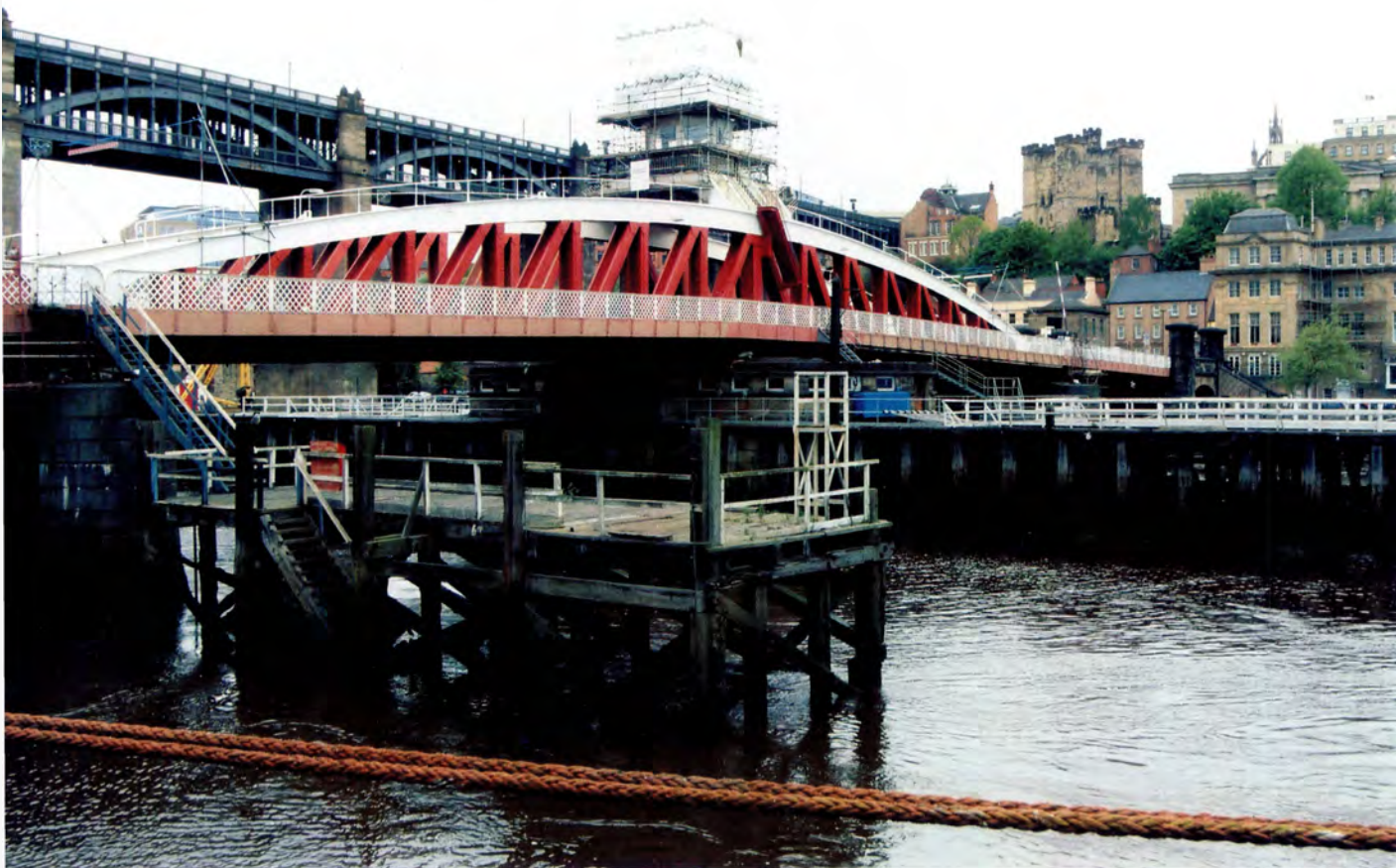
Fig 1 The swing bridge of 1868–76, which replaced an earlier stone arched bridge, swings on a central axis to allow ships to pass. The keep of the castle, on the site of the Roman fort, overlooks the river crossing. [DP000124]
