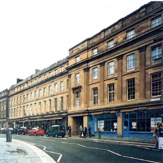
Fig 14 Grainger Street. The frontage to Grainger Market, made up of three-bay units designed to give a shop on the ground floor and living accommodation over. One of the 14 entrances to the market can be seen in this view. [AA040918]
