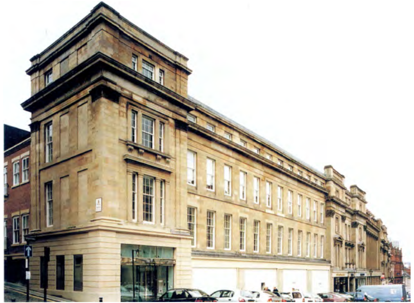
Fig 13 52–78 Grey Street. The use of pavilions to break up the terrace elevations helps to accommodate the fall of the land to the south. [AA040921]
