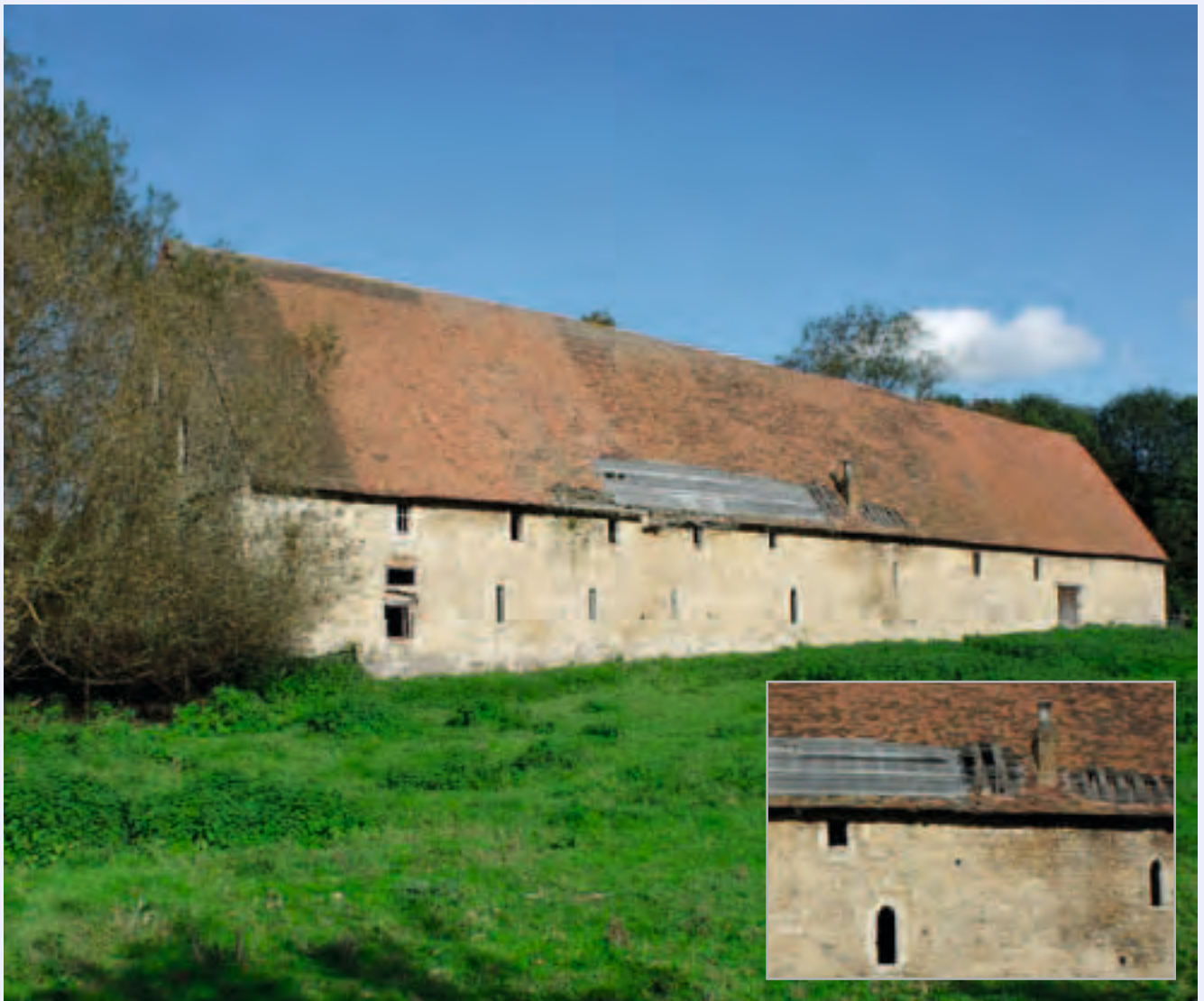
Boxley Abbey 'barn' in Kent (a scheduled ancient monument that was probably once the Abbey's hospitium). It was repaired in 2012 with financial input from English Heritage, English Nature and the Society for the Protection of Ancient Buildings. A low-key use is now planned by the owner. © John Bailey, SPAB
