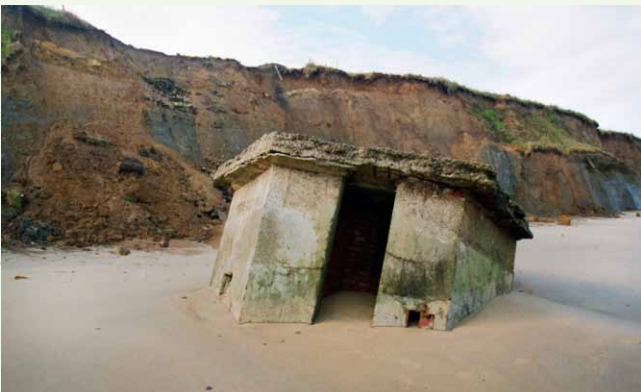
Second World War Pill Box facing coastal erosion at Happisburgh, Norfolk.
