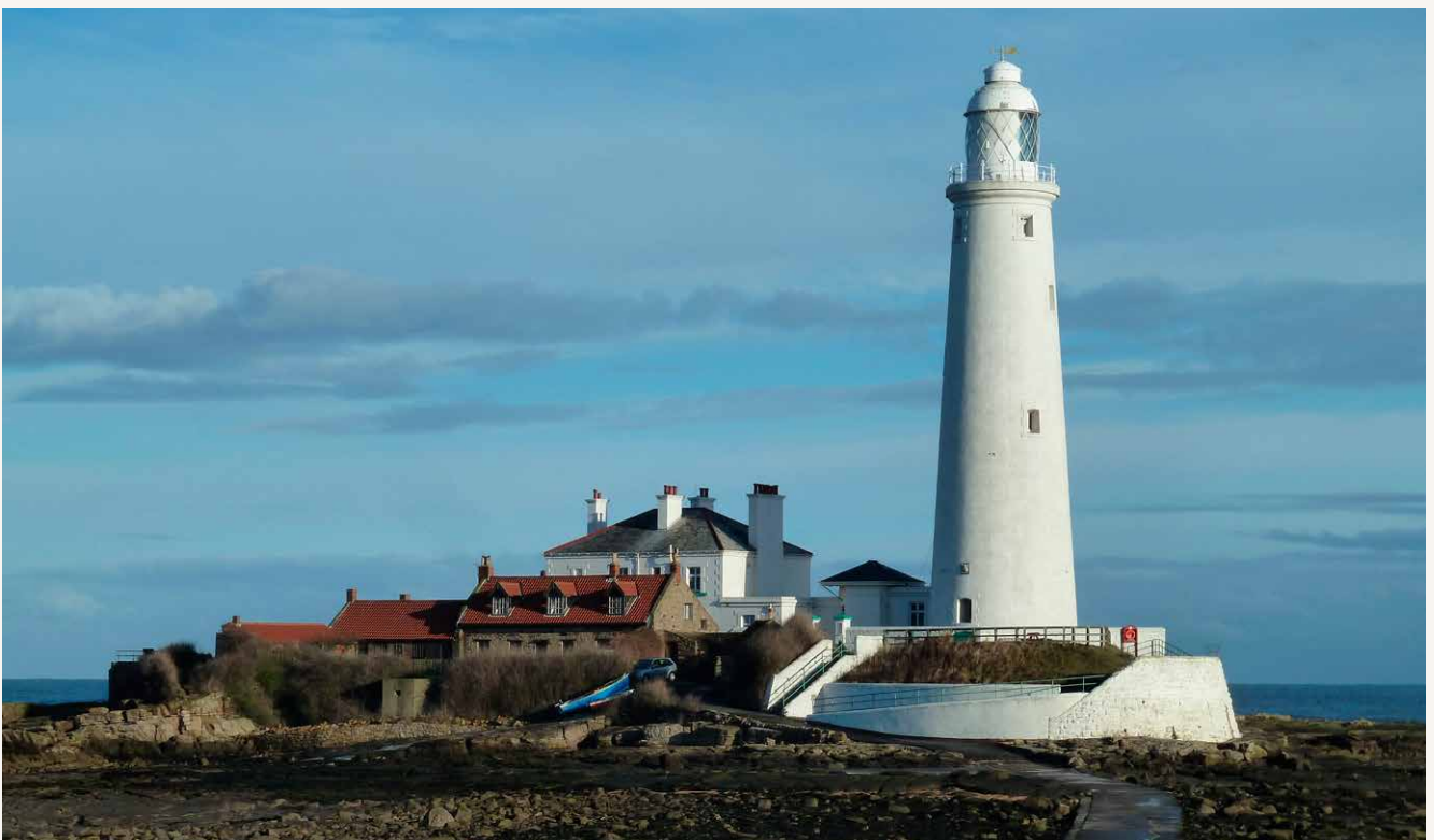
St Mary's Lighthouse and cottages, Whitley Bay, Tyne and Wear, Grade II (5A3) © Historic England
