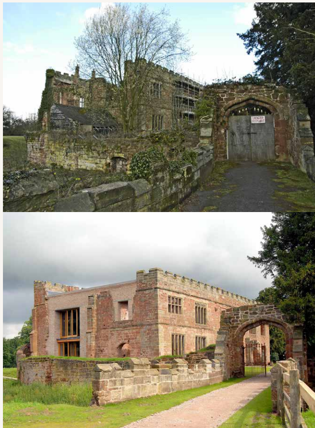
Astley Hall, Warwickshire, before restoration and after restoration (8A3) © Historic England
