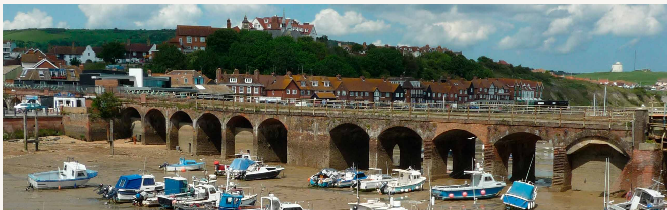
Folkestone harbour viaduct and swing bridge, Kent, Grade II (5A3) © Historic England
