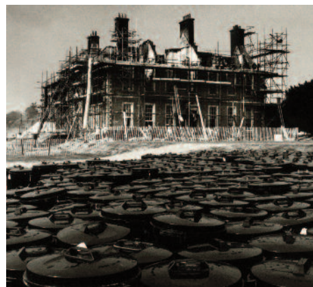
Figure 19 The fire damaged exterior of Uppark after the August 1989 fire, with dustbins for salvaged material. ©NTPL/Paul O'Connor
