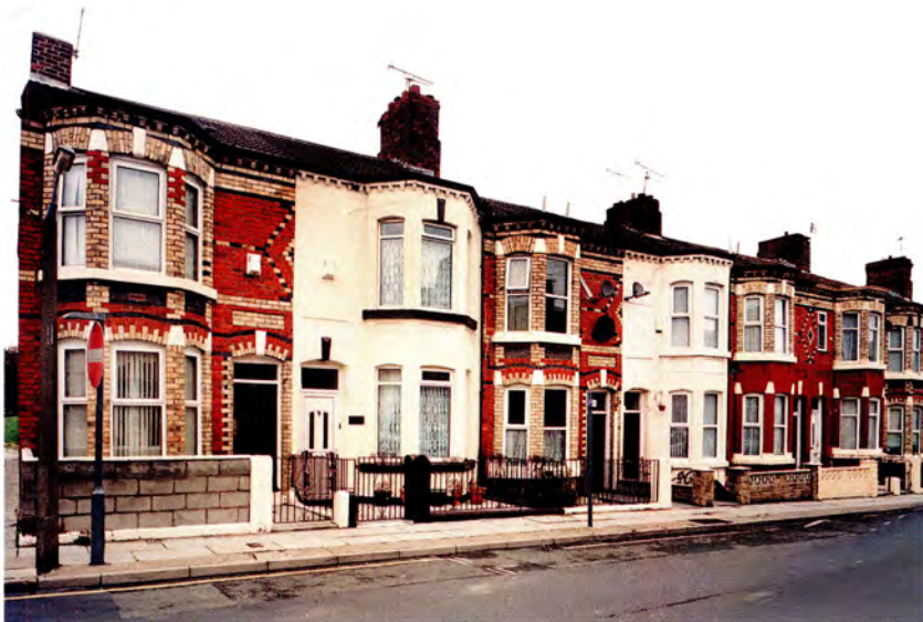
Figure 40 (above) 25 Arkles Road illustrates the range of mass-produced terracotta ornament available to the builder by the 1880s. The original iron railings to the forecourt walls are lost, but other details, including the panelled door and under-floor ventilation grille, remain. [AA045520]
