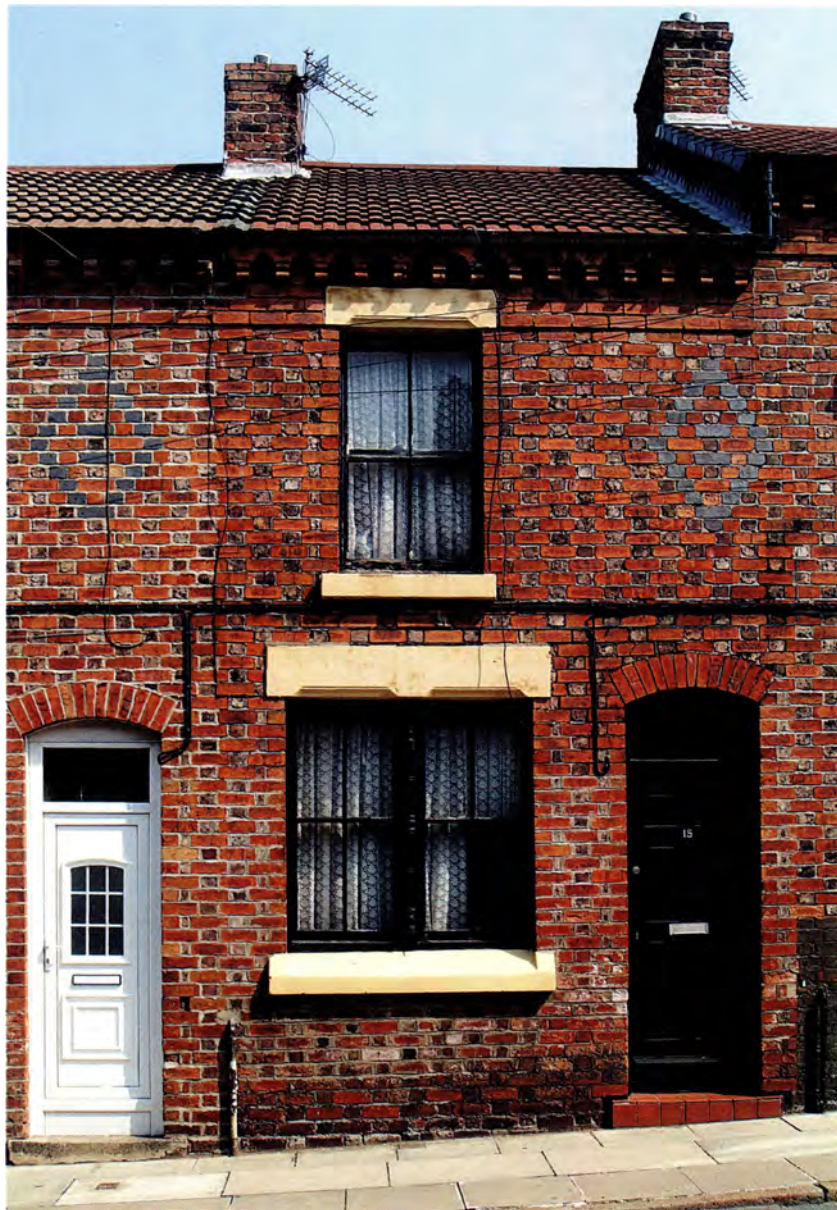
Figure 34 The smallest houses built in Anfield and Breckfield between 1860 and 1900 were of the two-up, two-down terraced variety, but all had elements of decoration. This example at 15 Saker Street has a brick diaper pattern and a moulded brick eaves course, whilst the paired sash is divided by a turned wooden mullion. These mullions, once common, are now increasingly rare. [DP027838]
