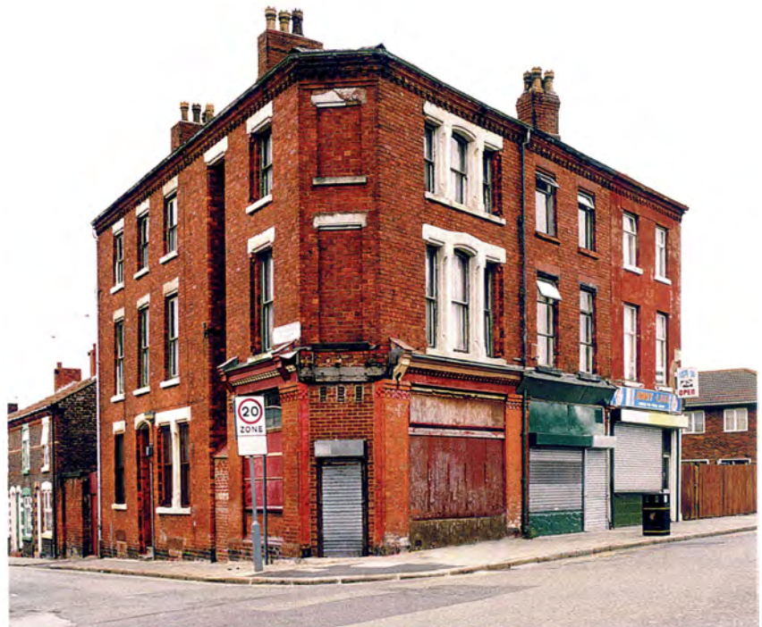
Figure 50 Nos 96, 98 and 100 Breckfield Road North, built c1885. No 100 (nearest), originally the premises of a bread-and-flour dealer named Richard Taylor, has a long taking-in slot in the left-hand wall for receiving goods on the upper floors. [AA045107]
