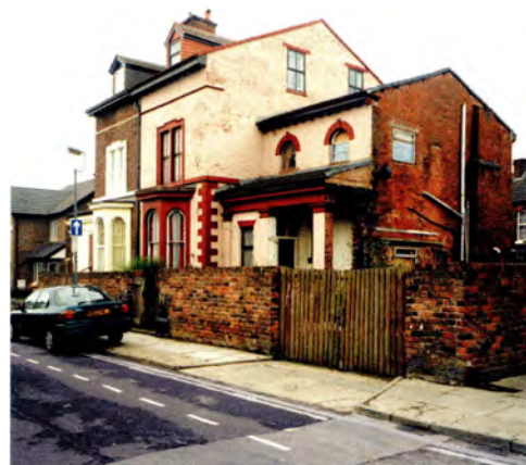
Figure 22 The size and aspect of the villa plot led to variations in design: (a) (left) at 21 and 23 Anfield Road (1870s) unusual apse-like sculleries are placed on the entrance front in order to keep the more prestigious garden front (overlooking Stanley Park) clear; (b) (above) 90 and 92 Burleigh Road South (c1870) occupy shallow plots and consequently place services, as well as the entrance, in a side projection. [AA045478, AA045546]
