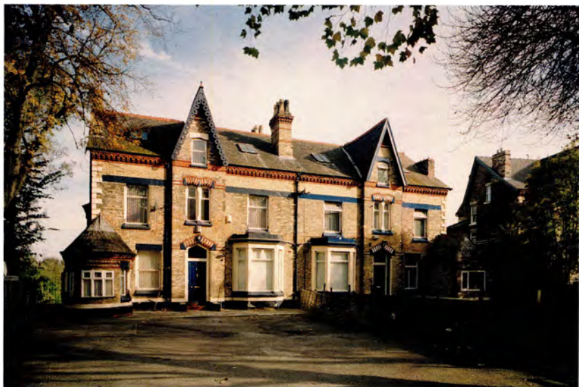
Figure 22 The size and aspect of the villa plot led to variations in design: (a) (left) at 21 and 23 Anfield Road (1870s) unusual apse-like sculleries are placed on the entrance front in order to keep the more prestigious garden front (overlooking Stanley Park) clear; (b) (above) 90 and 92 Burleigh Road South (c1870) occupy shallow plots and consequently place services, as well as the entrance, in a side projection. [AA045478, AA045546]
