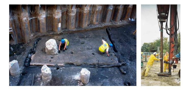
Figures 11 and 12: Sheet pile retaining wall along the edge of a site at Drapers' Gardens (left) © Pre-Construct Archaeology Ltd. Rolled steel tube being installed at Skirbeck Road, Boston (right). Steel pile installation is covered in detail in guidance provided by the Steel Piling Group (2018).
