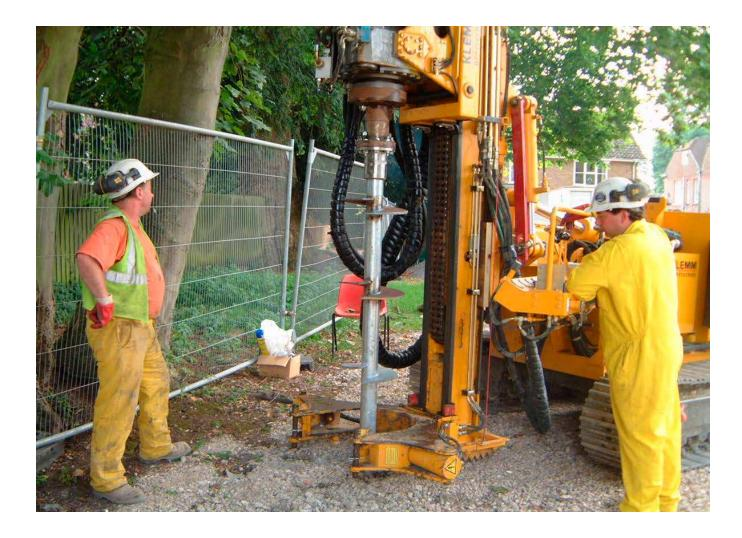
Figure 36: Screw piles being installed. © Tim Sheward
