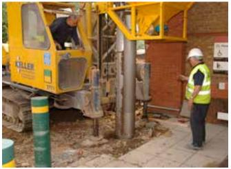
Figures 19, 20, 21: Bottom feed vibro replacement. © Keller Ground Engineering
