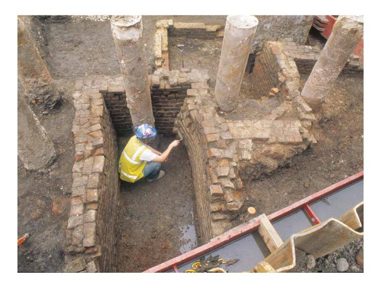
Figure 31: Piles can be located to avoid structures identified in evaluation or a site strip. © MOLA
