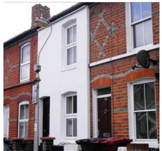
An insensitive external wall insulation application which damages the beauty and character of the whole street.
