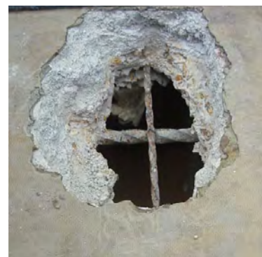
Reinforcement sampling and low reinforcement cover to soffit
