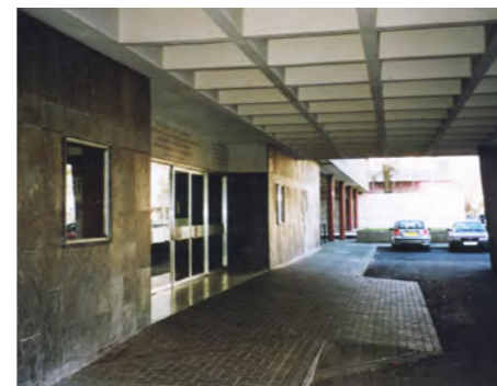
The porte cochere entrance
