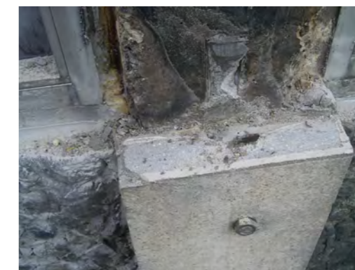
Non-ferrous metal pilaster restraint fixing
