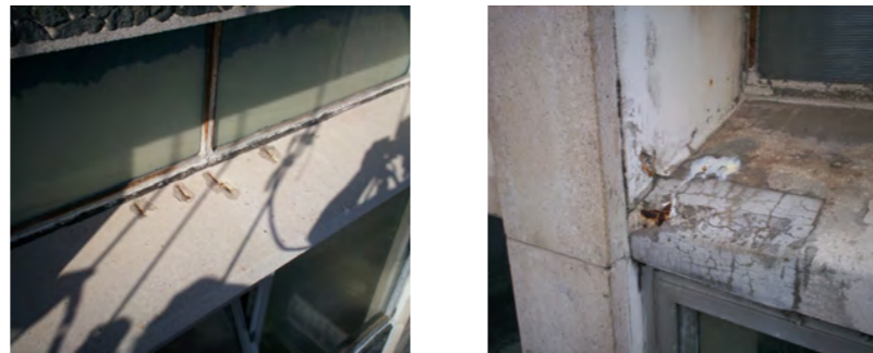
Pre-cast concrete transom cills
