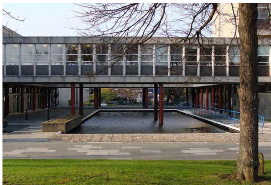
Continuity of landscaping from Armada Way through to the courtyard pool
