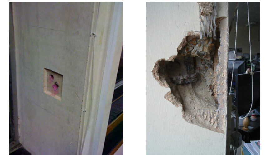
Chloride dust sampling and carbonation testing (left). Reinforcement inspection (right).
