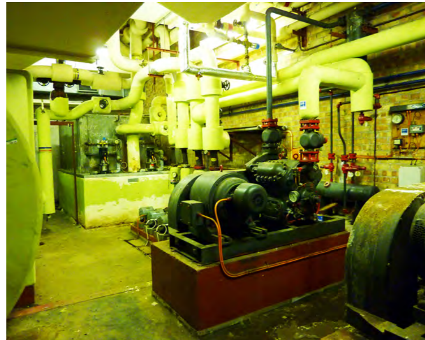
Redundant refrigeration plant
