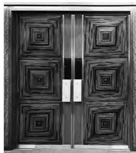
Raised doors of courbaril
