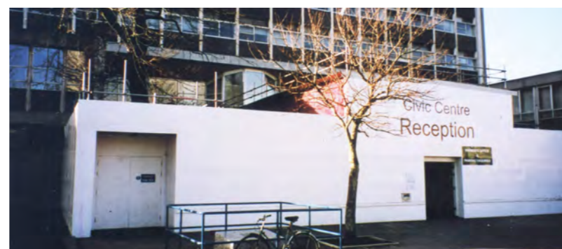
Entrance enclosure now
