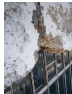
Corrosion in parapet at movement joint. Side view (right). Top view (left).
