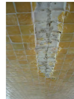
Cracking in second floor soffit - area knocked out to expose extent of cracking
