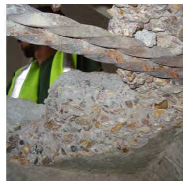
Reinforcement sampling and low reinforcement cover to soffit
