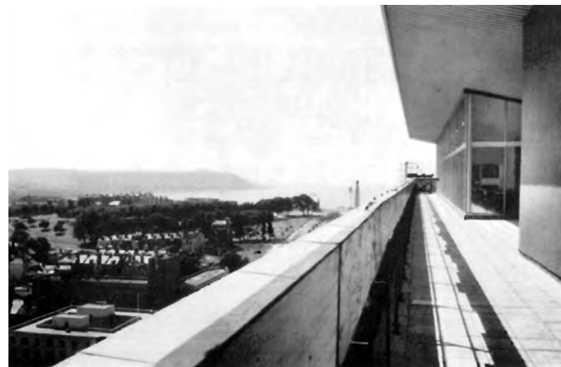
Roof terrace, original
