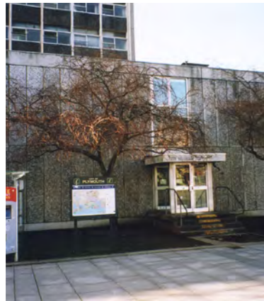
New entrance to north block
