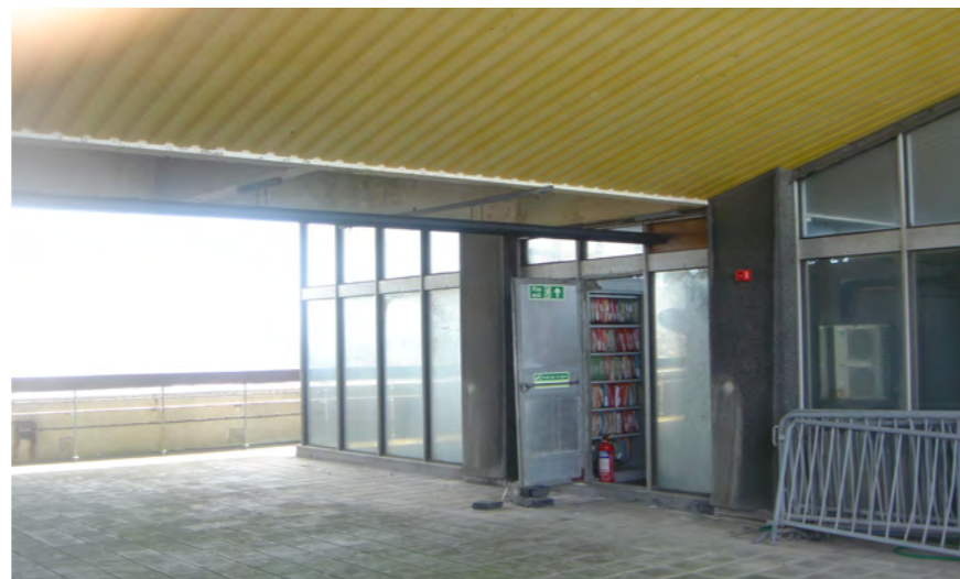
Roof terrace, current
