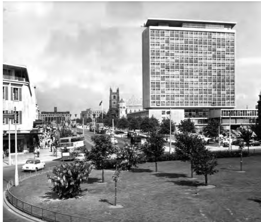
Middle distance view of tower with its façade pattern
