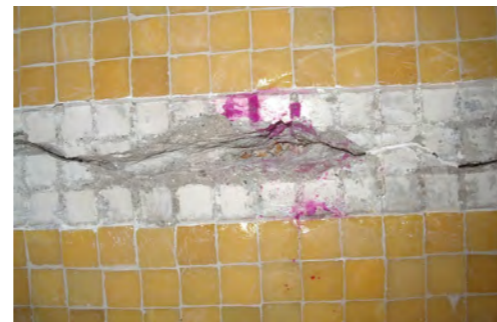
Cracking in second floor soffit - area knocked out to expose extent of cracking
