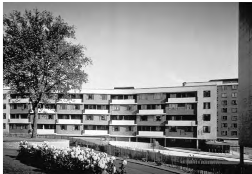
Spa Green Estate, London 1950 - one of many dynamic façades by Berthold Lubetkin
