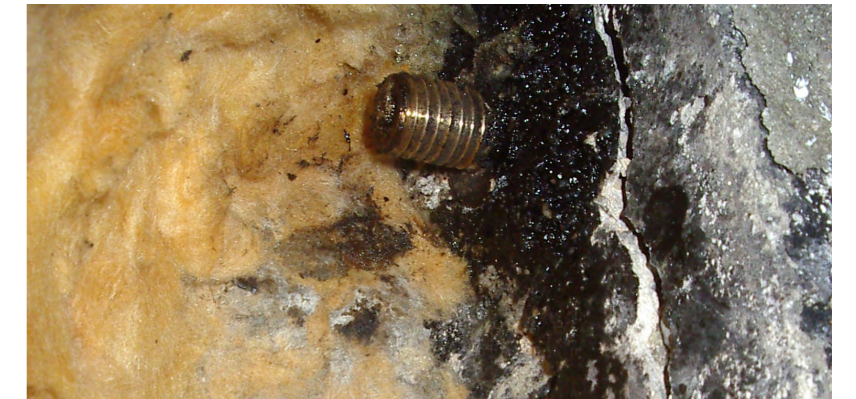
Non-ferrous spandrel panel bolt fitting
