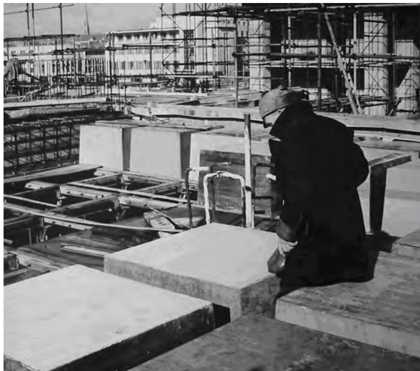
Timber formwork for waffle slabs
