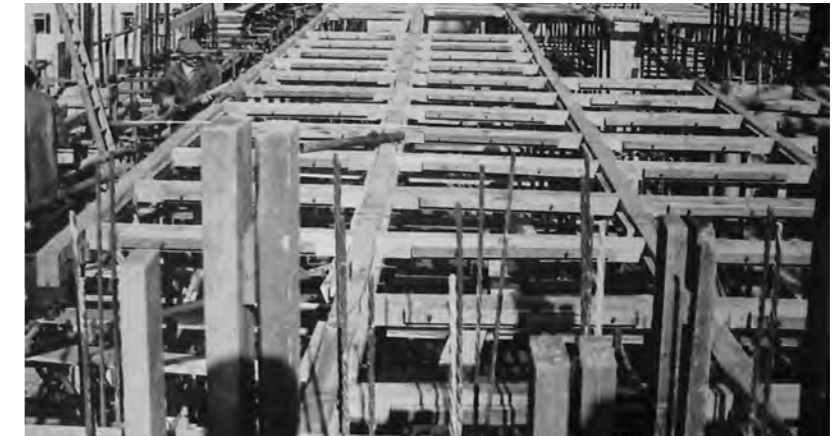
Column reinforcement projecting above slab. Continuous between floors
