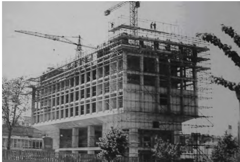
Second floor load transfer slab visible during construction
