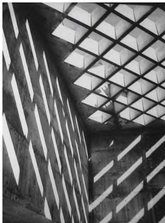
Exposed structural framing of diagonal grid rooflight during construction
