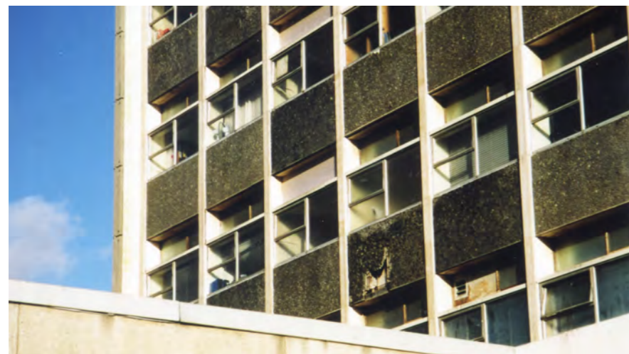
Close up of window details, current
