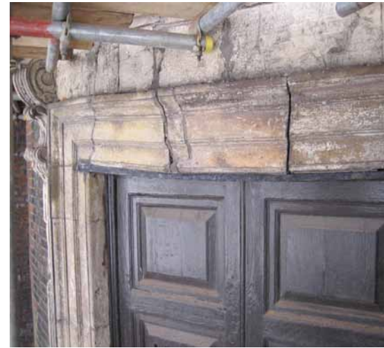
St George's Theatre in Great Yarmouth showing original and replacement fine scroll brackets, a failing stone lintel repaired in situ, and new and original brickwork © David Grech.
