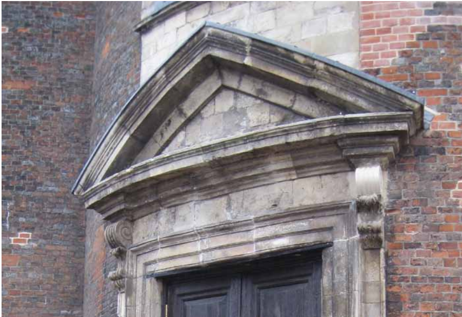
St George's Theatre in Great Yarmouth showing original and replacement fine scroll brackets, a failing stone lintel repaired in situ, and new and original brickwork © David Grech.
