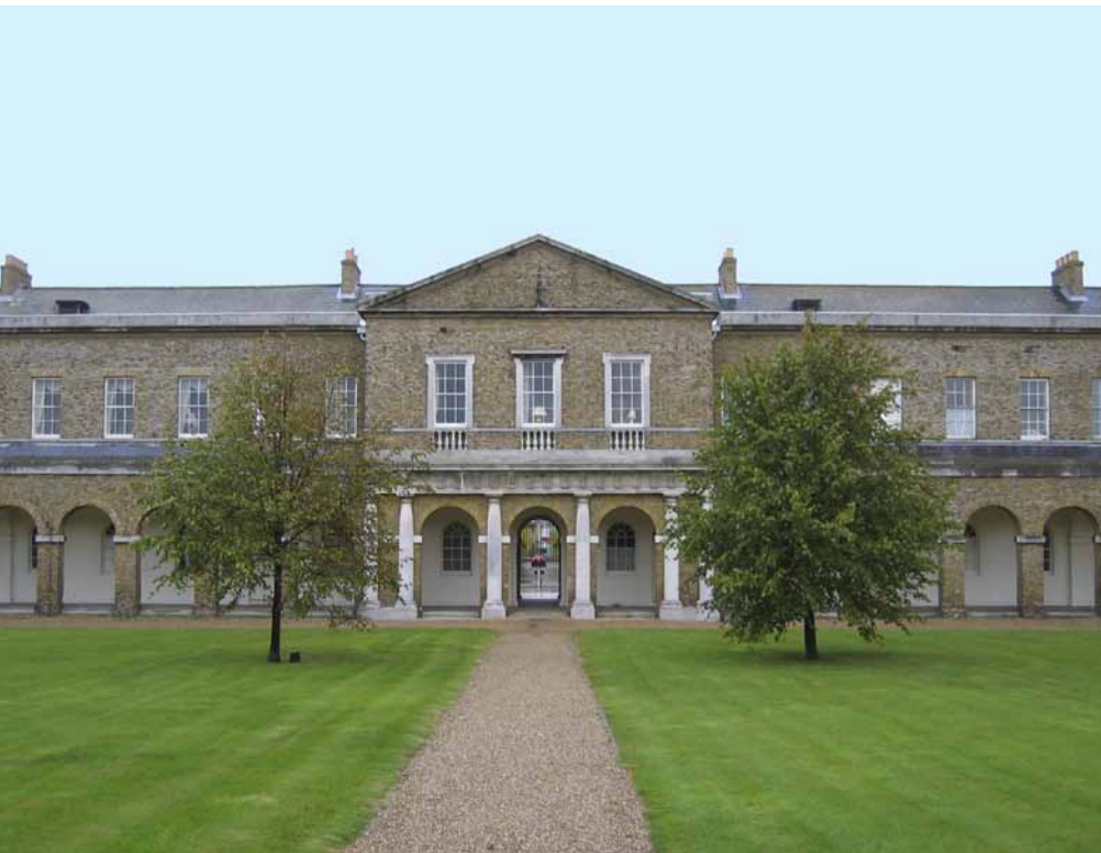
The grade II* former Naval Hospital at Great Yarmouth which has been converted into apartments and houses © David Grech.
