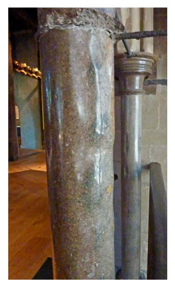
**Figure 30 (left):** Deteriorated material has been removed and the surface polished, but this has left the column with an undulating topography that is very obvious in reflected light.
