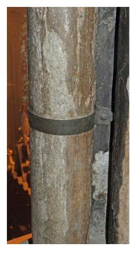
**Figure 28 (above):** An example of using a copper band to provide medium to long-term security for a column at Ely Cathedral. Signs of cleavage are evident.
