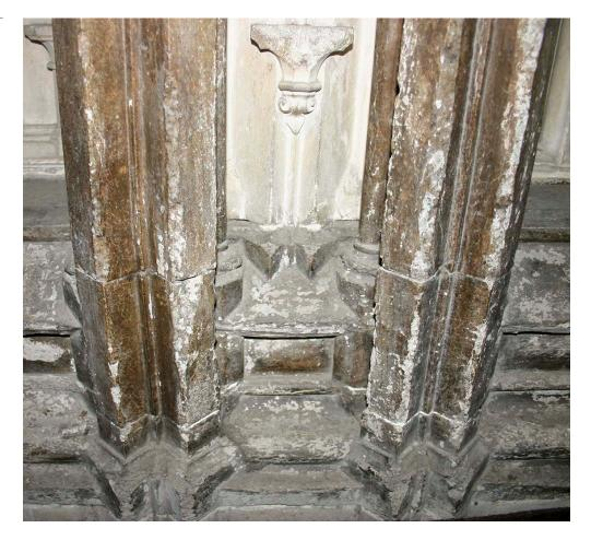
Figure 22: A monument to Edward II (1284-1327), dating from the 1330s, in Gloucester Cathedral. Low-level abrasion and surface deterioration due to combination of visitor action and rising moisture.
