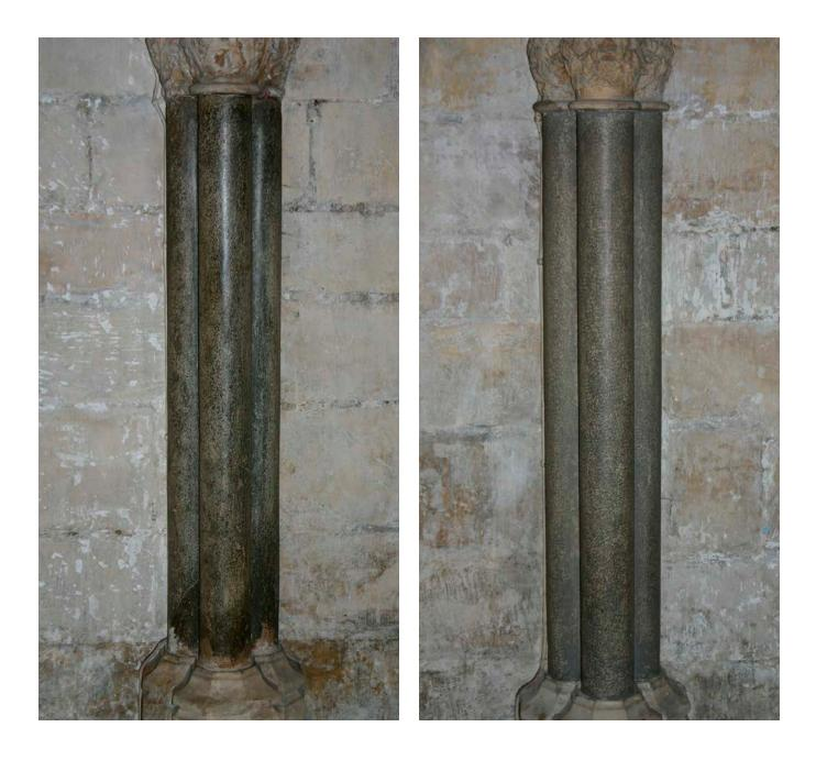
**Figure 33:** Zouche Chapel, York Minster: a polished Purbeck Marble column cluster (left) and replacement Bath Stone column cluster painted to look like Purbeck Marble (right). The painted stone has a good colour match, but lacks the depth of sheen which a polished Purbeck Marble surface provides.
