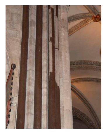
**Figure 25 (left):** Scagliola repairs at Canterbury Cathedral were applied to match the dark brown surface of the Purbeck Marble as a result of discolouration of a wax surface coating. However when the surface coating was removed, the repairs now appear in stark contrast to the original pale colour.
