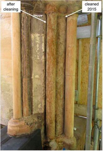
**Figure 39:** At Norwich Cathedral cloisters, the heavily soiled and coated columns were cleaned using a poultice of synthetic latex and EDTA. Dwell time had to be carefully controlled to avoid over cleaning and all the poultice material had to be removed using dry steam.
