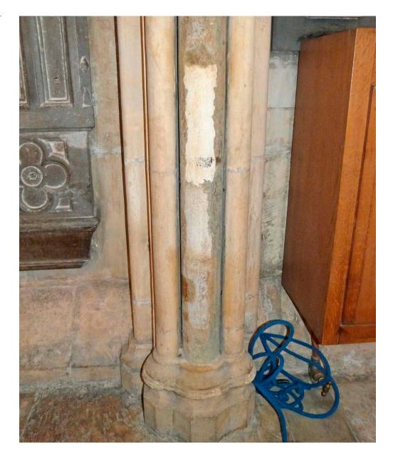
**Figure 40:** Removal of surface coatings can often reveal previous repairs beneath. These in the north choir aisle at York Minster may be inappropriate either in appearance or composition and will need to be re-done. Suitable methods for removal are generally based on dissolving the coating. Solvents can be organic or inorganic. The choice will depend on the nature of the surface coating and the desired result. Possible materials include:
