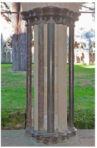
**Figure 49:** A new Purbeck Marble column and capital in Norwich Cathedral cloisters. The surface has been given a honed finish rather than polished. Microcystalline wax has been applied as a protective finish. **Figure 50:** A new Purbeck Marble column in Salisbury Cathedral cloisters inserted and treated with pigmented wax.
