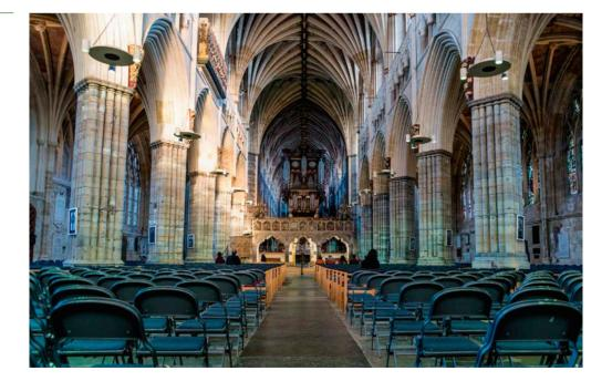
**Figure 41:** The Purbeck columns in Exeter Cathedral nave have been cleaned of dirt and surface coatings and left untreated. The complete removal of surface coatings can make Purbeck Marble appear pale and sometimes bland. It is usually good practice, particularly in fluctuating environmental conditions, to apply appropriate new treatments to both protect the stone and improve its appearance.
