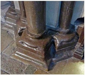
**Figure 31 (above):** A Purbeck Marble column base in Canterbury Cathedral reworked (in the 1930s) to remove decayed material and then polished. The surface is now sound but the detail of the form has been lost.
