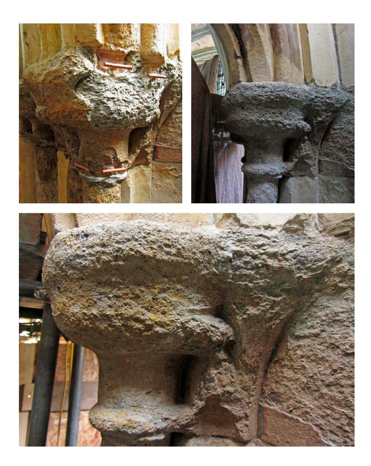
**Figure 47:** Repairs to Purbeck Marble capitals in Norwich Cathedral cloisters: (top left) A Purbeck Marble capital prepared for repair with loose material removed and ceramic armatures in place. (top right) Repairs of a Purbeck Marble capital completed using mortar based on lime putty. (bottom) Repairs to a Purbeck Marble capital completed with pigments blown onto the surface.
