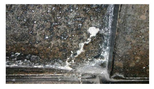
**Figure 18:** Localised damage due to sub-surface crystallisation of salts on the side panel of a medieval monument.
