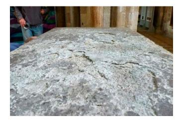
**Figure 45:** The top of a chest tomb at Chichester Cathedral before (above) and after (right) consolidation of spalling Purbeck Marble with dispersed lime injection mortar.
