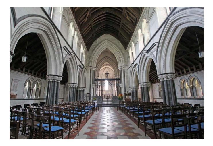
**Figure 7 (above):** At St James' Church, Kingston, Dorset, Purbeck Marble has been used for columns, abaci, string courses and hood moulds to provide contrast with the pale Portland Stone ashlar and arches.
