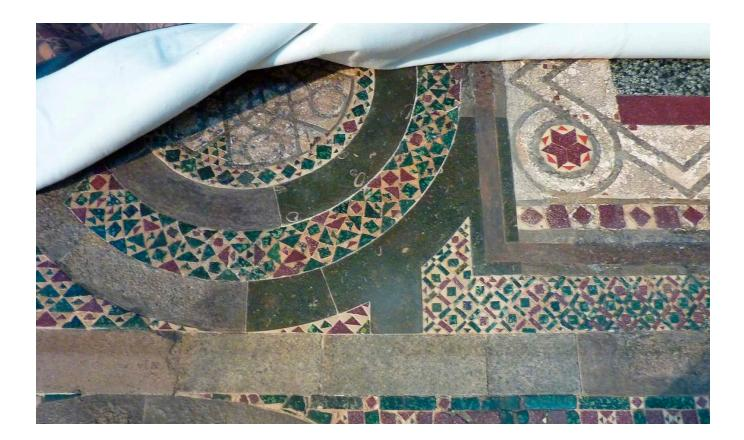
**Figure 51:** Insertion of new Purbeck Marble into the framework of the Cosmati pavement at Westminster Abbey.
