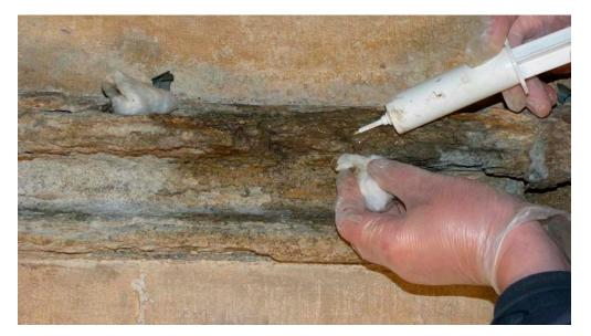
**Figure 44:** Using dispersed lime injection mortar (mixed 1:1 with trass) to secure spalls of an internal Purbeck Marble string course at York Minster. Although the texture of an eroded Purbeck Marble surface can be replicated using selected aggregates, matching colour is far more difficult. However, recent work at a number of locations has shown that sensitive application of pigments to the surface of lime mortar can successfully mimic the overall appearance of Purbeck Marble.
