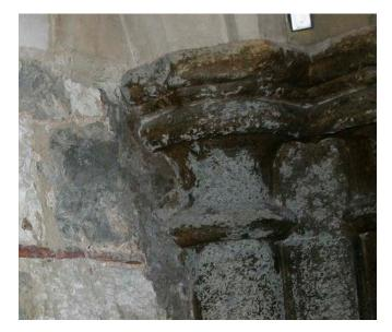
**Figure 20:** The deterioration of the wax coating here is a result of environmental factors. Fluctuations in humidity affect the stone behind the coating leading to the deterioration of both.
