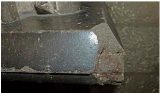
**Figure 27:** An example of multiple repairs to a capital in Norwich Cathedral cloisters using perhaps three different mortars, none of which provide a good aesthetic match. Note the unrepaired capital behind.
