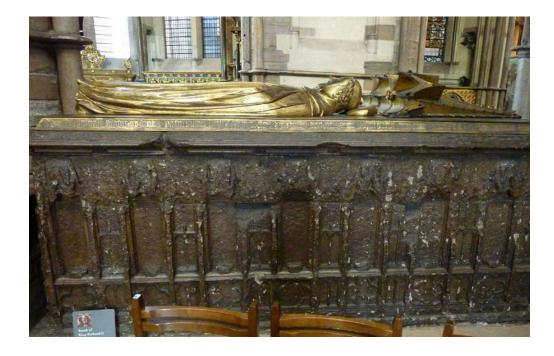
**Figure 5:** The monument to Richard II (1367–1400) and Anne of Bohemia (1366–1394) in Westminster Abbey is constructed from large slabs of Purbeck Marble set on edge. The nature of the stone means that carving is intricate but does not have fine detail. Discolouration is due to a conservation treatment, known as 'induration', applied in the 19th century.
