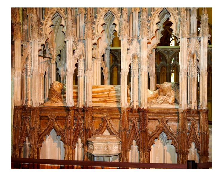
Figure 11: A monument to Edward II (1284–1327), dating from the 1330s, in Gloucester Cathedral. The base is carved from Purbeck Marble in exquisite detail. The dark brown appearance is due to discolouration from repeated applications of beeswax.
