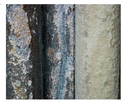
**Figure 43:** Completed grouting of a split in a column in Salisbury Cathedral cloisters.
