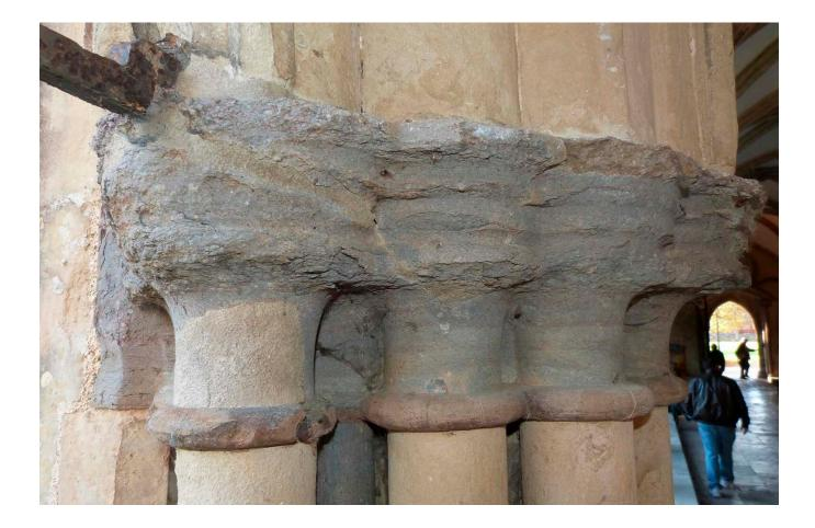
**Figure 34:** Capitals of a column cluster in Salisbury Cathedral showing a variety of issues including ongoing decay, poor previous repairs and (repaired) damage from the expansion of an iron bar.
