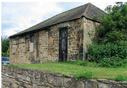
on the line, was entered via a turntable into the end elevation (*see* Fig 32). The Newcastle & Carlisle Railway shed at Fourstones (1838) (Fig 11) may also have been of the parallel type.
