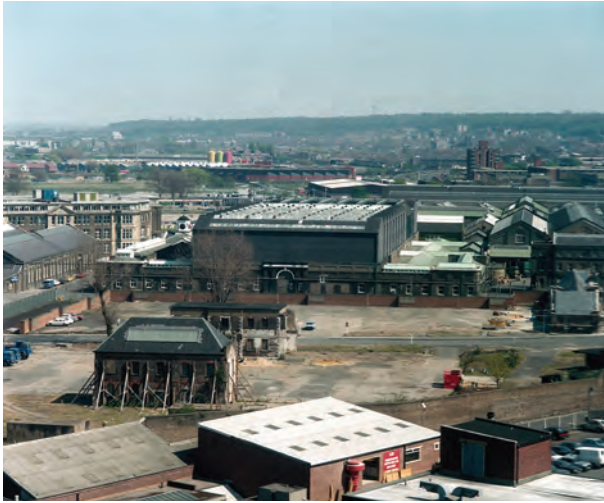
The former Carriage Department, one of the many major historic buildings on the Royal Arsenal, Woolwich, site. © BHL
