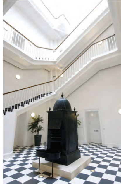
Right: The restored stairwell within Building 37, Royal Arsenal, Woolwich. © BHL
