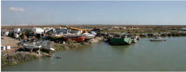
A scrap-metal yard on the site of the former dock alongside the Real Carenero, Cadiz. © UCA
