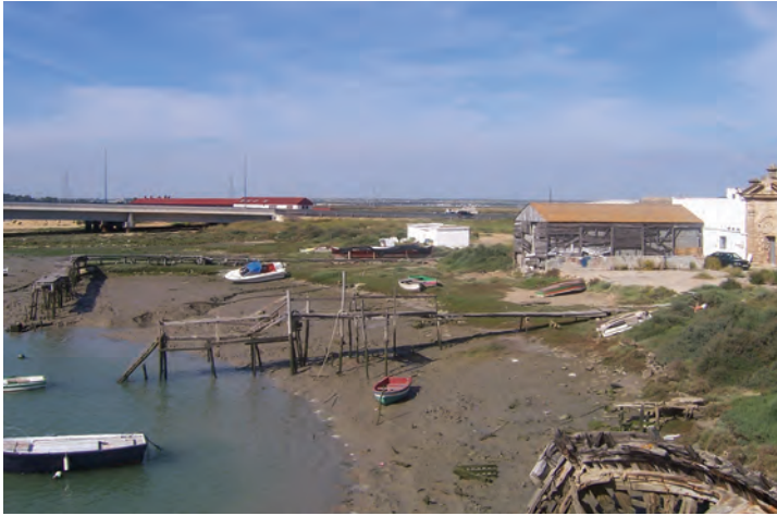
The Real Carenero viewed from Suazo Bridge, with the new road and bridge in the middle distance. © EH
