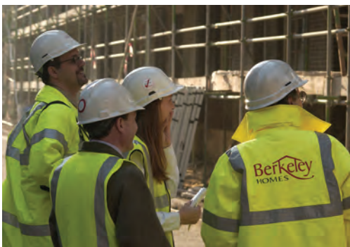
Staff from Berkeley Homes Ltd overseeing building work at the Royal Arsenal, Woolwich. © BHL
