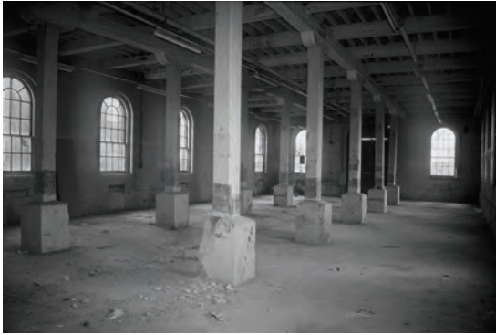
Interior view of one of the floors in the Grand Store, Royal Arsenal, Woolwich, showing the scale of the spaces available for conversion into residential units. © OA
