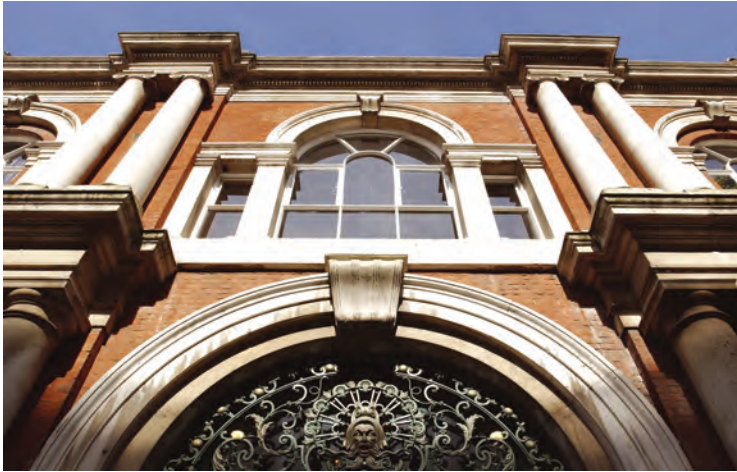
The Shell Foundry Gatehouse, one of the important surviving buildings within the Royal Arsenal, Woolwich, site. © BHL
