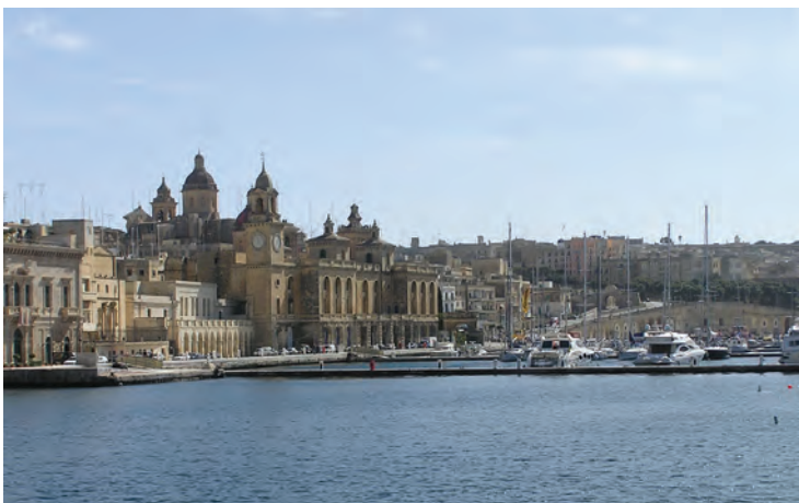
Vittoriosa Wharf, Grand Harbour, Malta. The central waterfront building now houses the Maritime Museum. © EH
