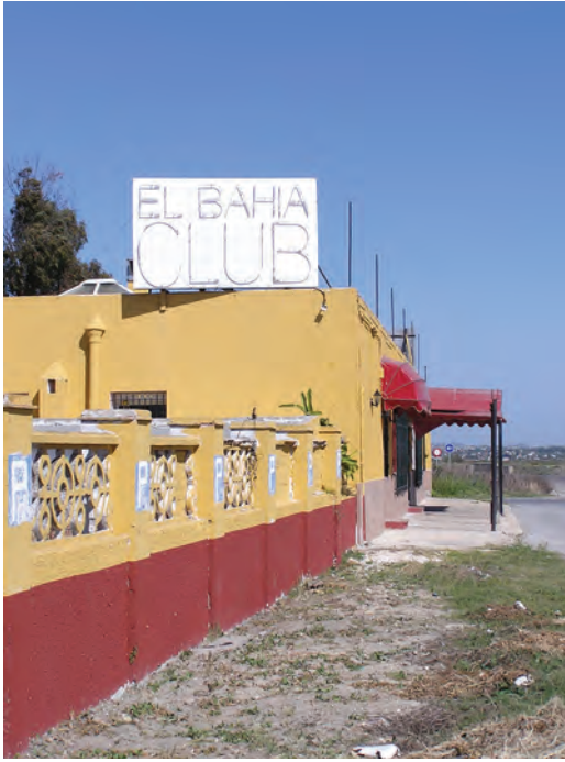
Occupying part of the Real Carenero site is a 'house of ill repute' that takes advantage of being on the boundary of different local authorities. © UCA
