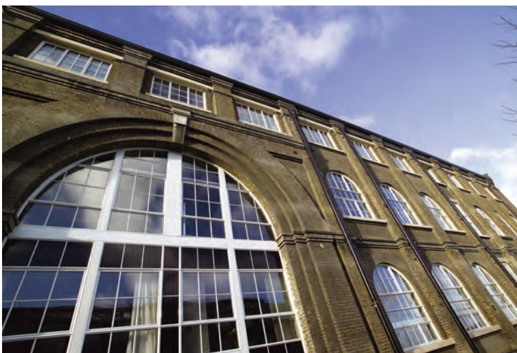
The restored exterior of one of the Grand Store buildings, Royal Arsenal, Woolwich. © BHL
