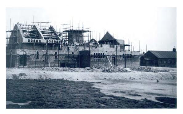
F L Charlton also designed St Cross, Middleton, and this view taken in 1935 shows how it was constructed using a series of concrete arches. To the right may be seen the temporary building that preceded it, typical of how many suburban churches started life. (Courtesy of St Cross)
