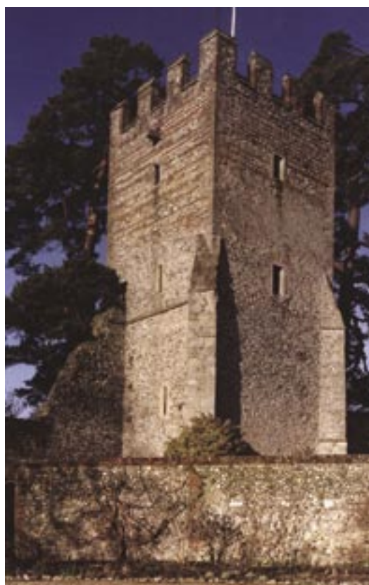
'The Great Tower': one of the medieval towers built by the Lords of Rotherfield. The upper stages were rebuilt during the post-medieval period
