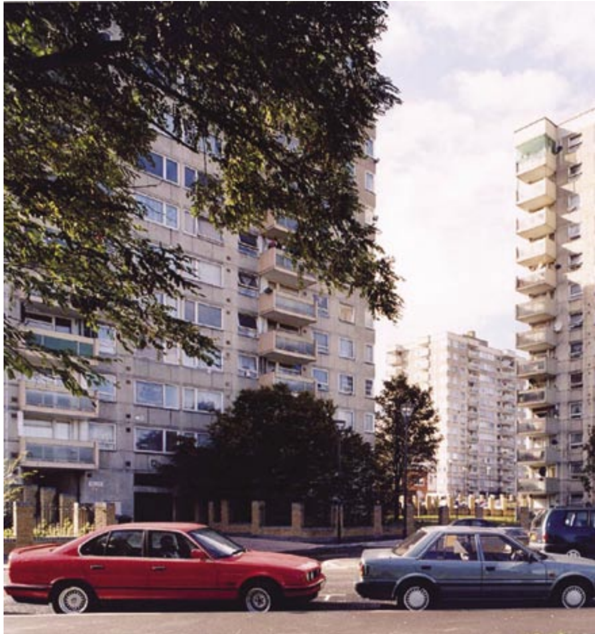
Fig 3. Corfe, Harlech and Beaumaris towers, three 13-storey blocks containing 228 flats, known locally as 'the Castles', 1968-71. Built for the London Borough of Ealing
