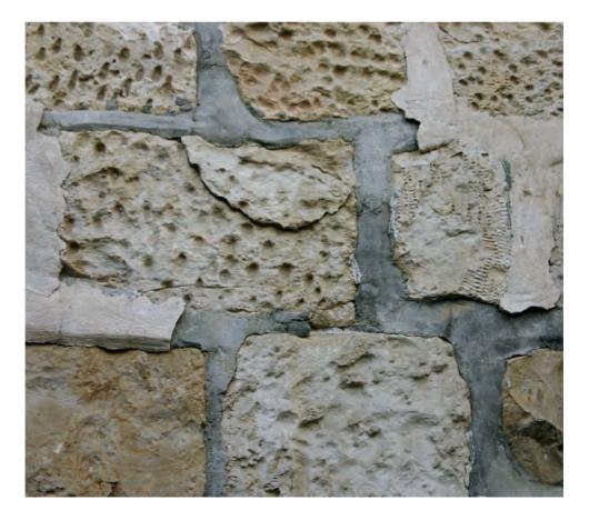
Pointing is often replaced unnecessarily when the original mortar is still sound
