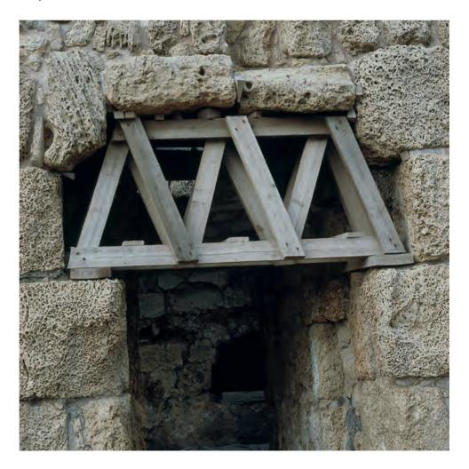
Decayed or missing jambs, lintels or mullions may require temporary support, either to allow further investigation or as part of the repair process. This is best done with timber struts or pins supported on either side of the opening. Helical ties or twisted wires can be inserted into a horizontal joint to tie across vertical cracks and act as a restraint for further movement.
