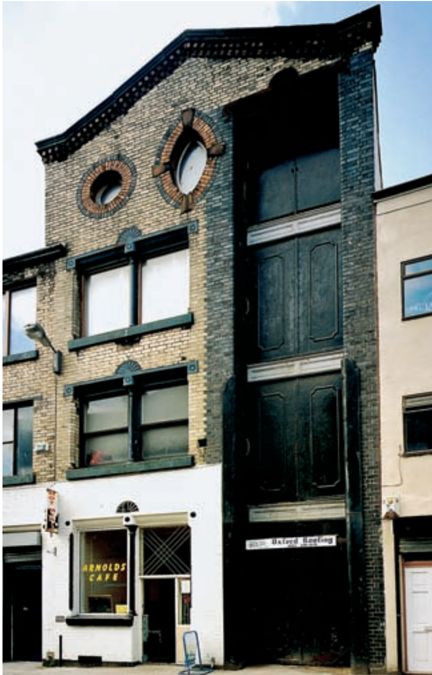
Fig 36 27 Cheapside: note the use of fireproof doors, large windows with cast-iron sills and lintels, and decorative polychrome brickwork. [AA045303]
