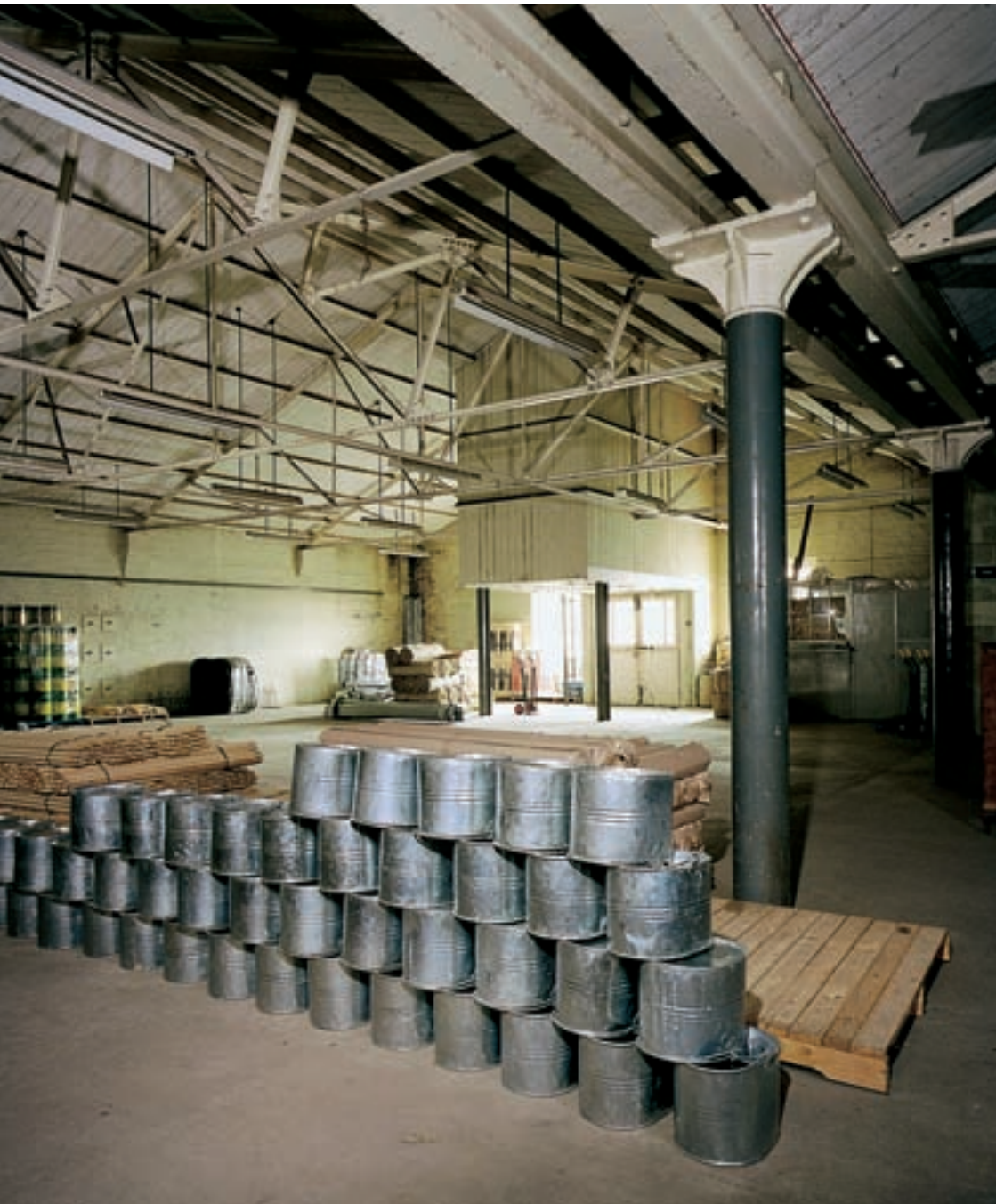
Fig 34 62-4 Kitchen Street, built in the early 20th century, has a wide span permitted by the use of light angle-iron roof trusses. [AA045301]
