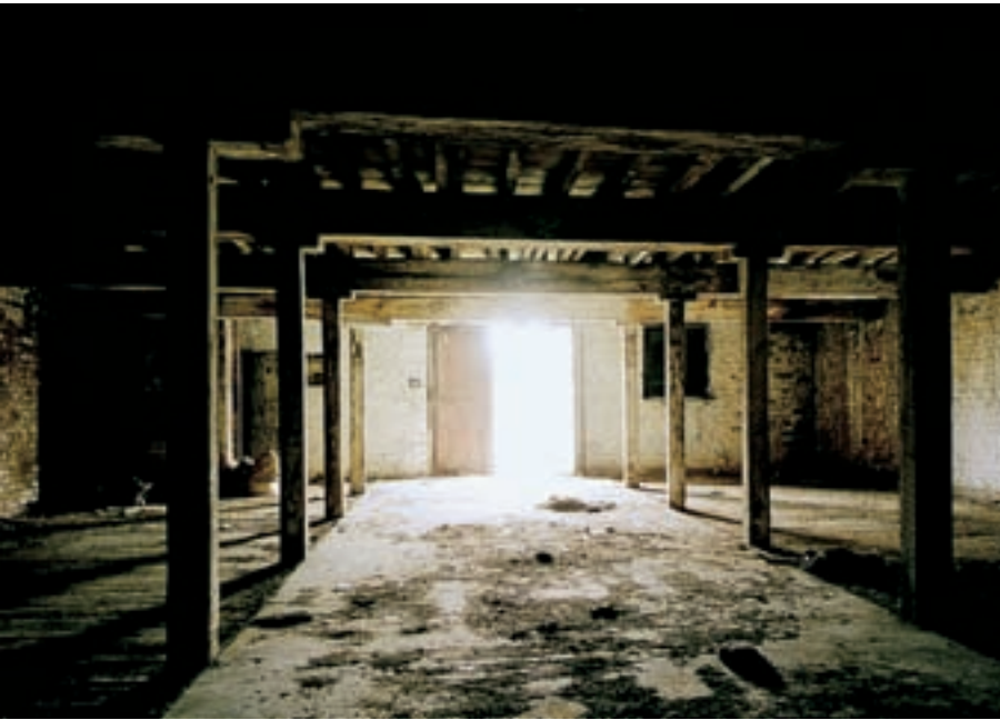
Fig 20 (opposite, top) The loading bay on the fourth floor of 46 Henry Street: the view shows the timber floor and timber prop. The rope harnesses hanging from the beam secured the warehousemen as they pulled goods into the building. [AA045279]
