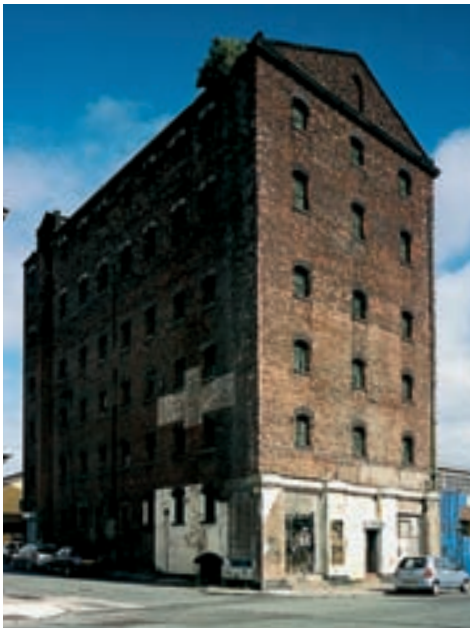
Fig 29 This warehouse at 68 Waterloo Road, at the junction with Vulcan Street, was probably built in the mid-1840s as a fireproof building. [AA045126]
