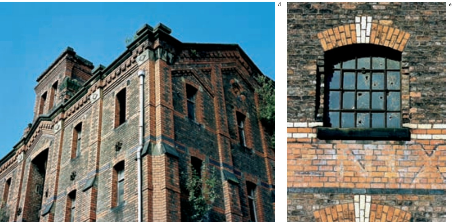
Fig 50 The character of warehouses. External details: (a) timber loading door and hoist beam at 22 College Lane [AA045314]; (b) iron loading door and hoist beam, Kitchen Street [AA045338]; (c) decorative brickwork at 45 Henry Street [AA045337]; (d) polychrome brickwork at 14–18 Henry Street [AA045336]; and (e) polychrome brickwork and metal window frame at Phoenix Oil Mill, Jamaica Street [AA045340].
