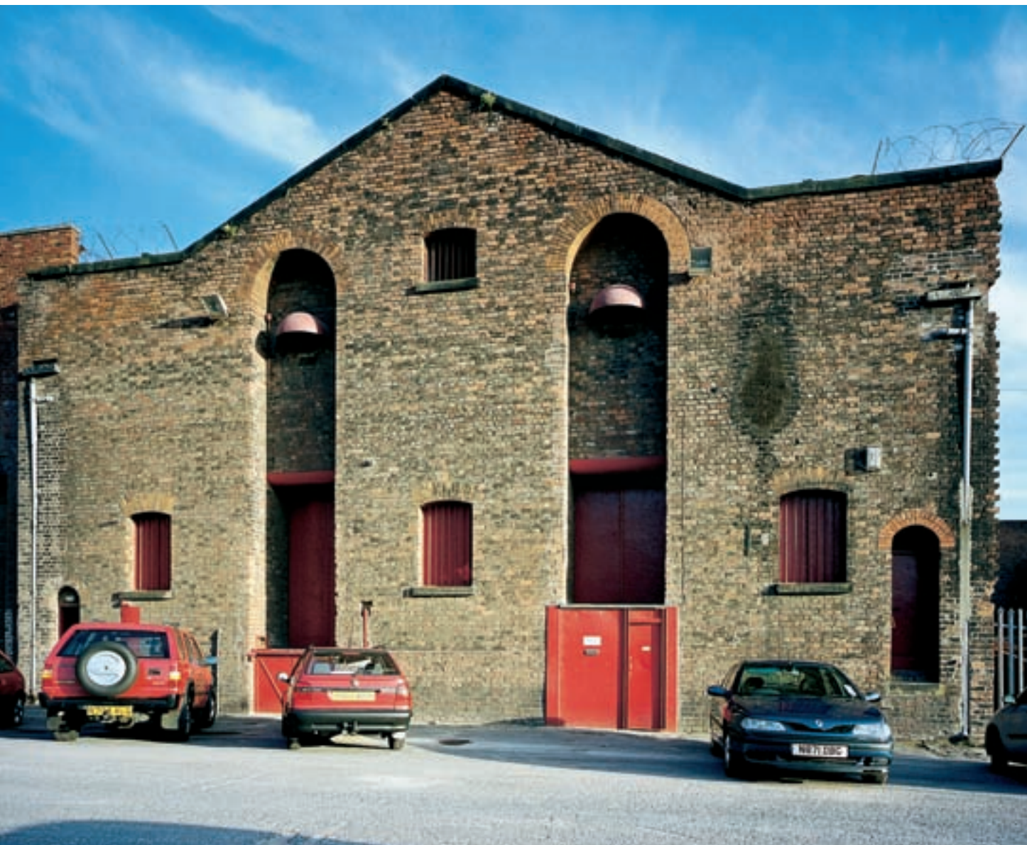
Fig 31 A low-rise warehouse at 8 Grundy Street: note how the loading bays have doors only on the raised ground floor. [AA045299]
