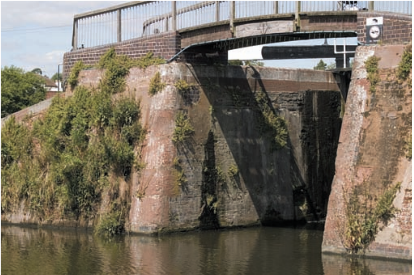
Figure 57 An example of erosion, wear and tear and potentially damaging plant growth on stonework and brickwork of canal structures. [DP022205]
