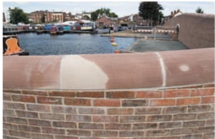
Figure 58 The new bridge on Mart Lane will allow boats to use the reopened Lichfield Basin (left); Coping from the parapet of the new bridge on Mart Lane: the use of traditional brick and natural sandstone ties in a modern structure to the historical pattern of materials in the town (right). [DP022194, DP022195]
