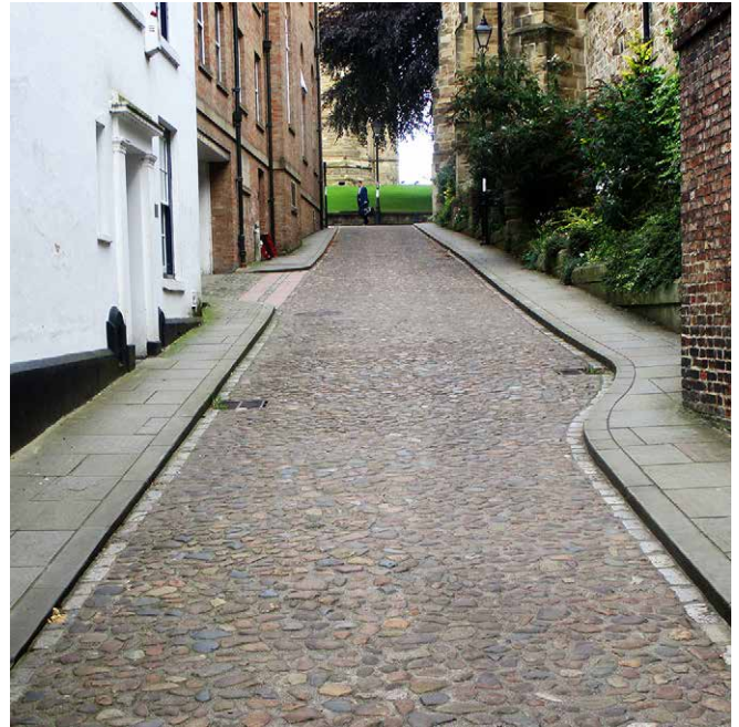
Bow Lane, Durham. This carefully re-laid cobbled surface provides a beautiful and durable lane in the historic heart of the city. As here, smooth paving should also be provided at crossings to assist users of wheelchairs or buggies. © Durham County
