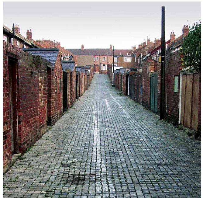
Traditionally, back lanes were laid with stone setts or blue scoria blocks, a by-product of the iron industry, and these survive in many areas, particularly across the Tees Valley.
